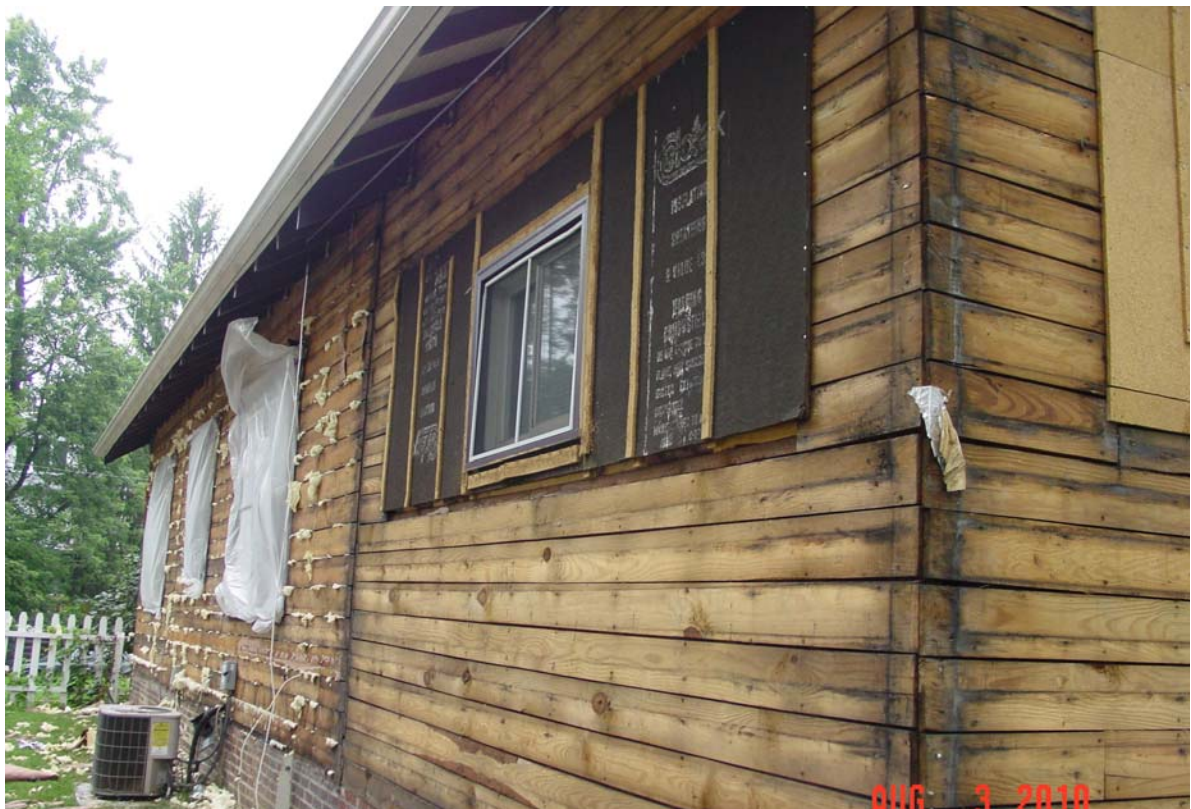
Below: View of East elevation of house. Markings are visible that show the original location and dimensions of the wood siding and trim.
