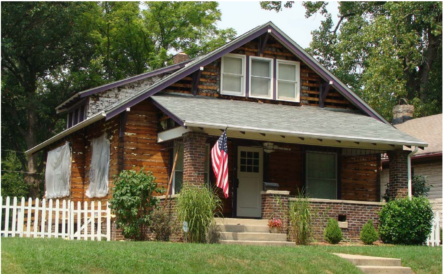
Above: Photo of house prior to removal of siding (with aluminum siding still on the house) Below: Photo of house after aluminum and wood siding were removed.
