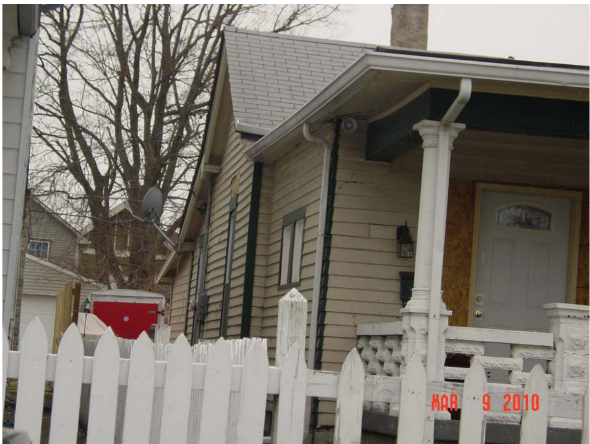
View of south side of house (and front porch in foreground)
