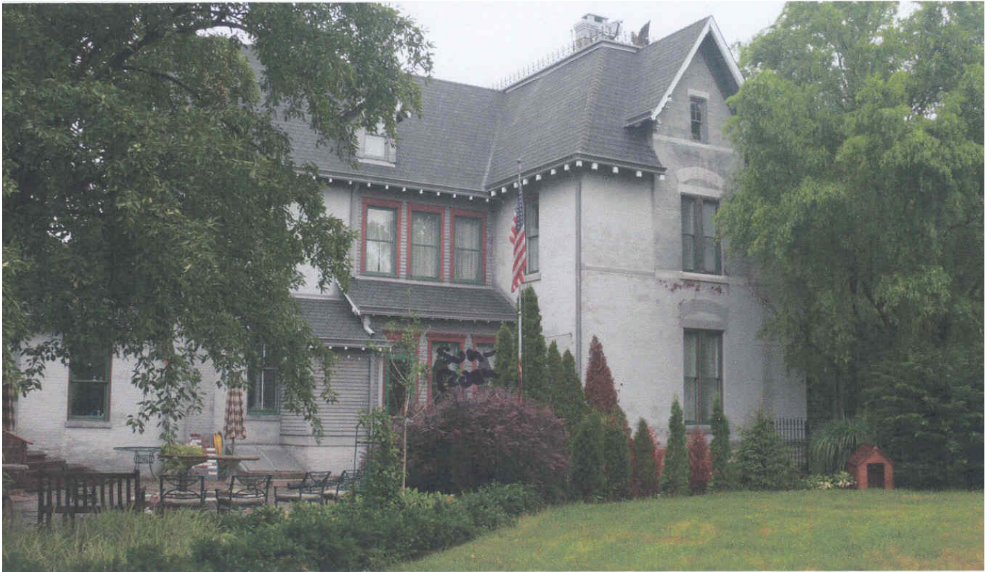
Above: Sunroom will be built on South elevation, extending south from shed-roof addition
