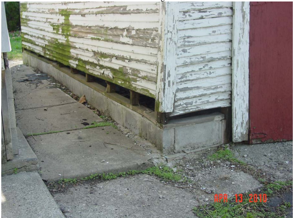
Detail of sill plate and wall studs
