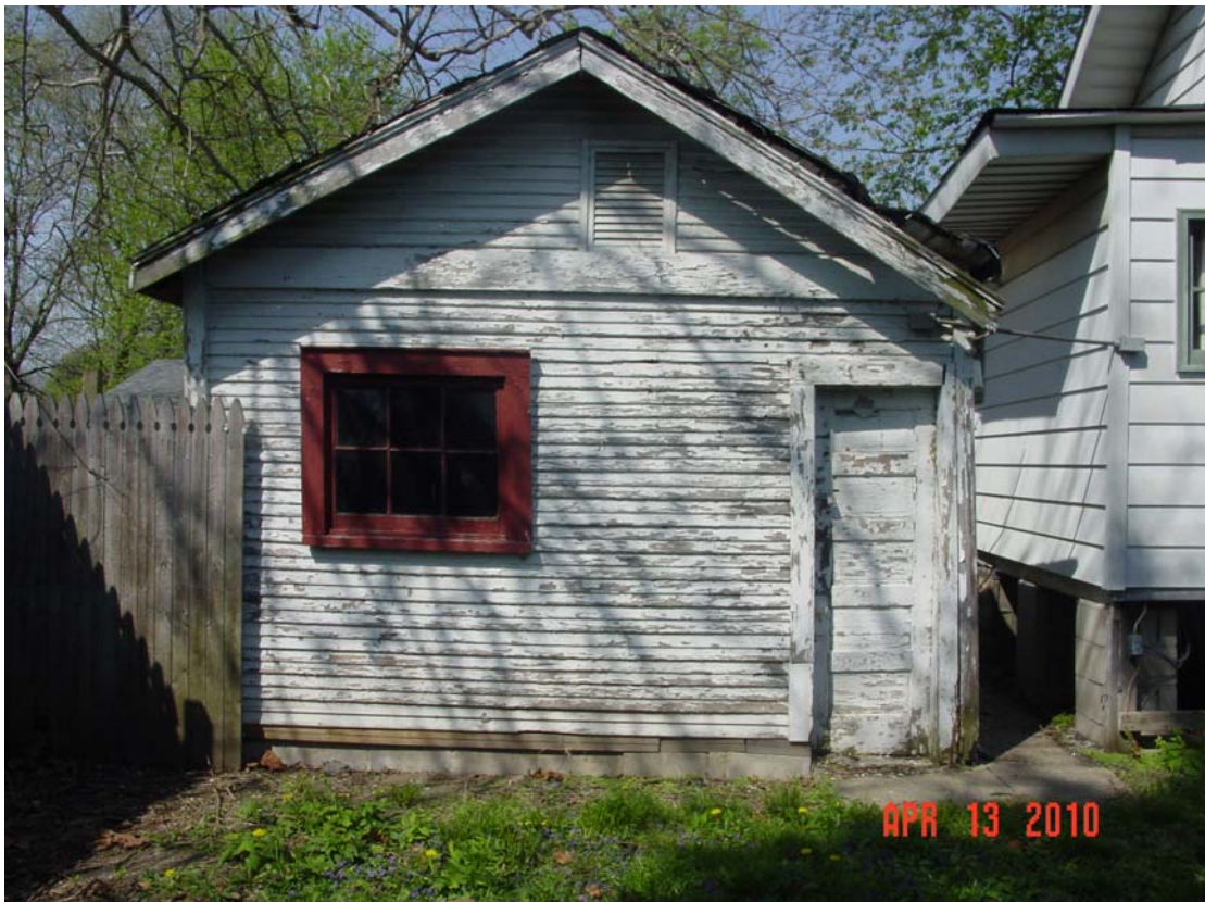
East side of garage
