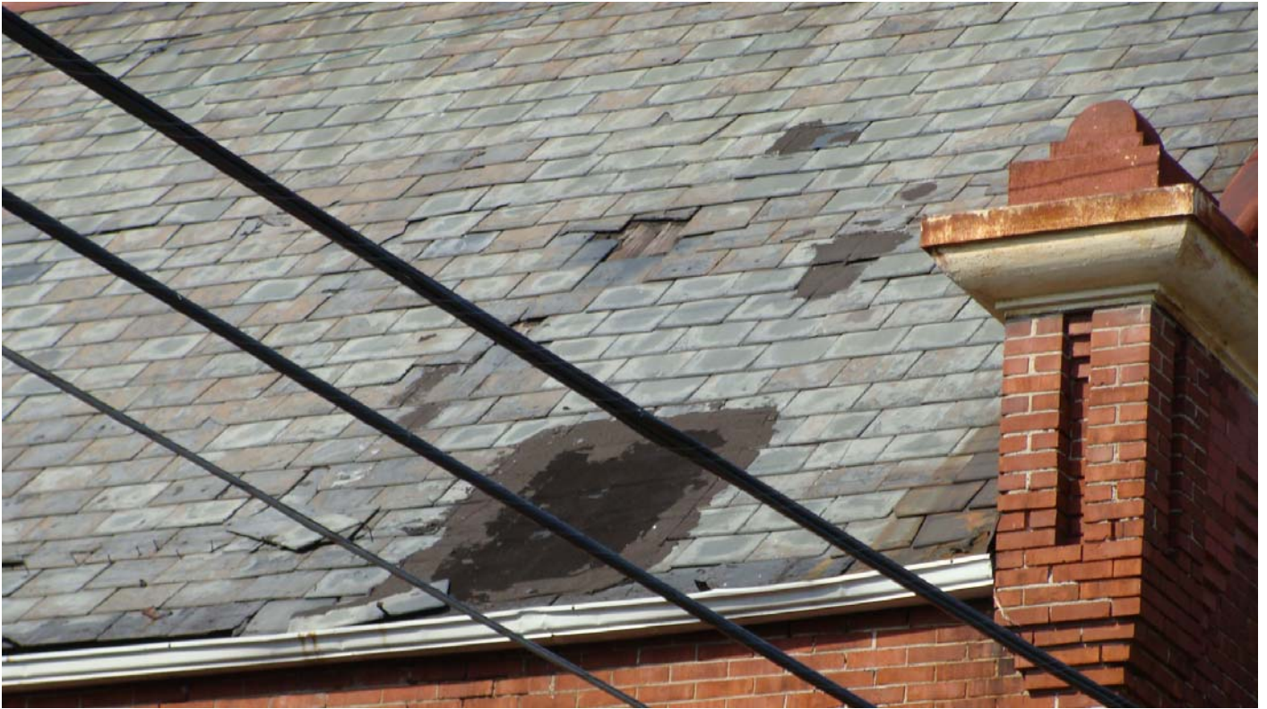
Detail of northeast corner of roof – looking southwest
