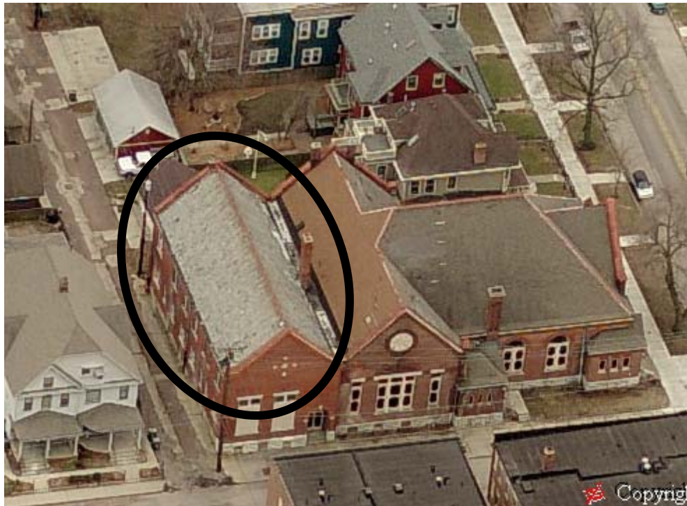
Aerial view of roof – looking south
