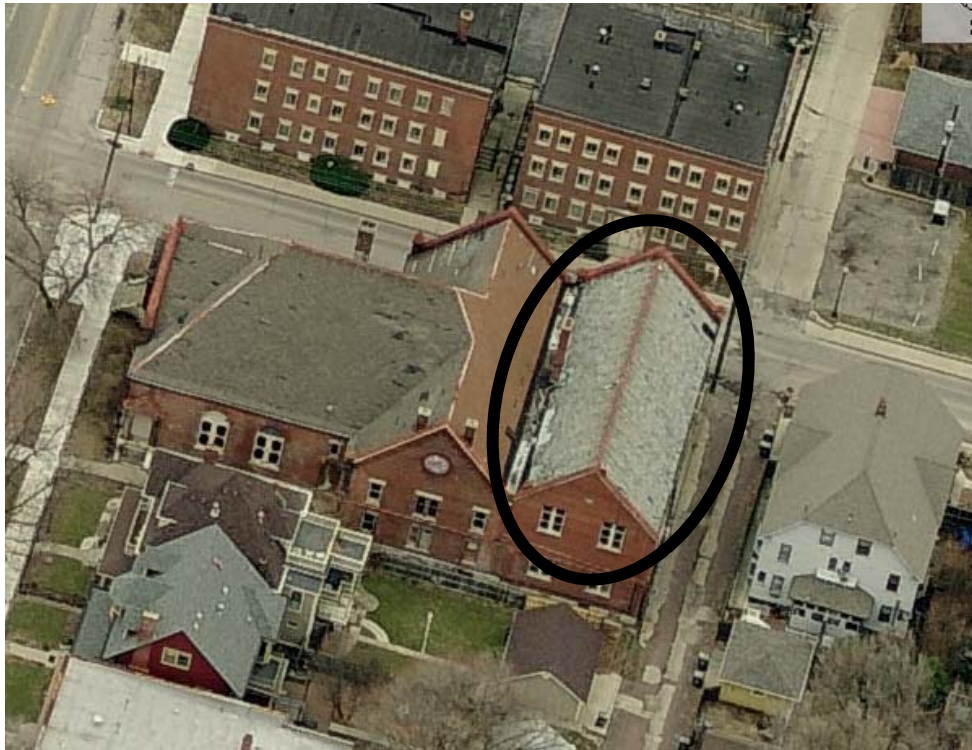
Aerial view of roof – looking north
