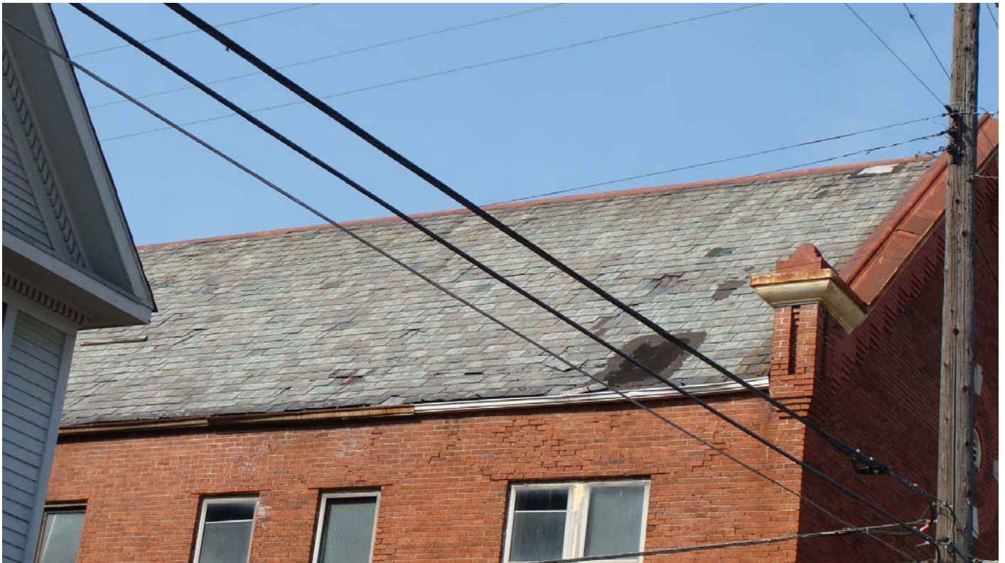
northeast corner of roof – looking southwest
