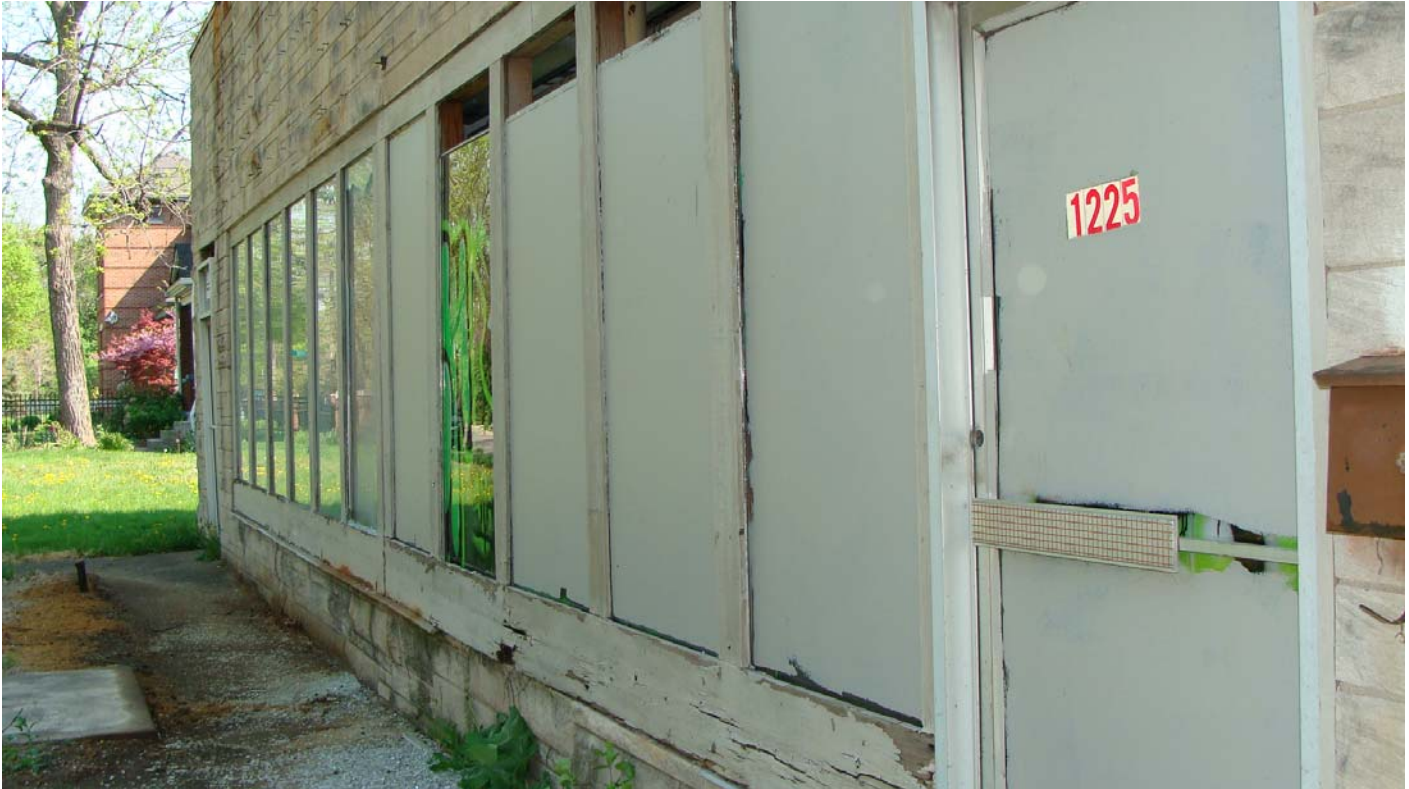
Close up of condition of front facade
