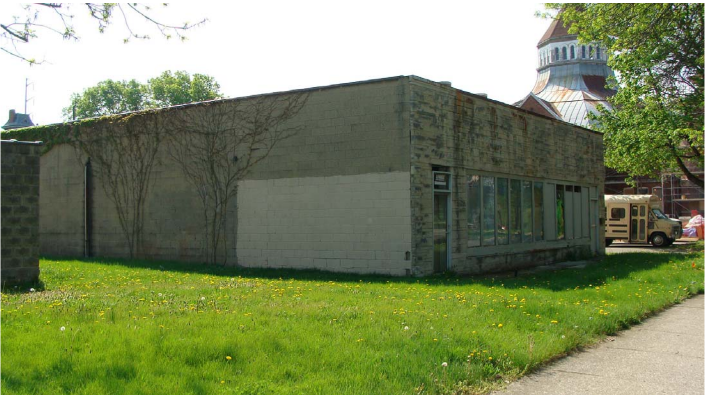
Photo of building looking south toward front facade
