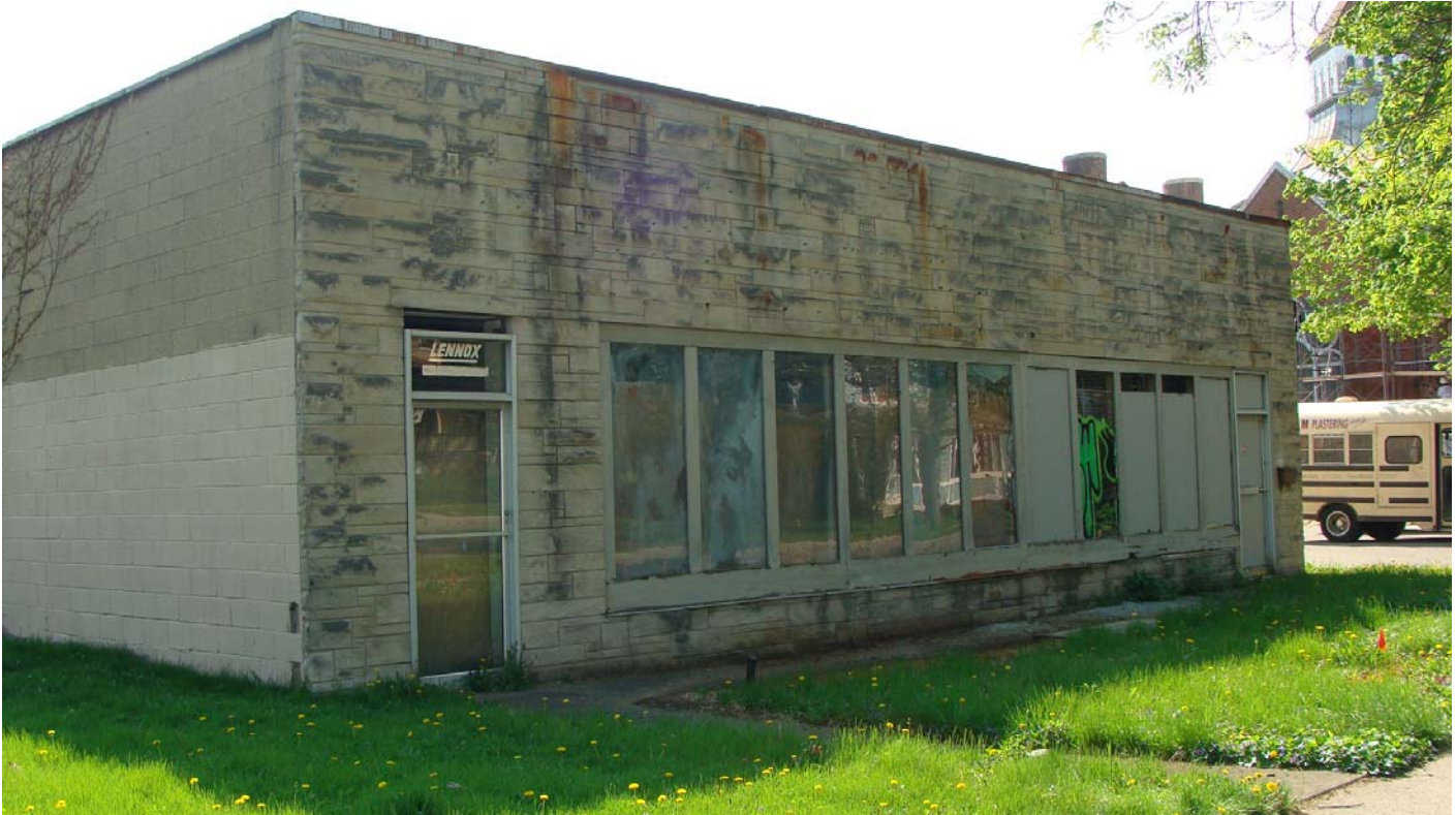
Photo of front façade (Storefront exhibits signs of modification over time)
