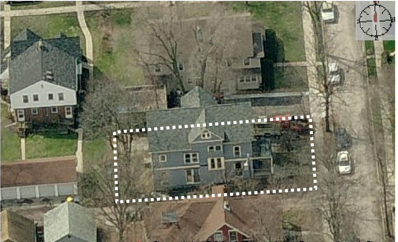
View of the property seen from the east
