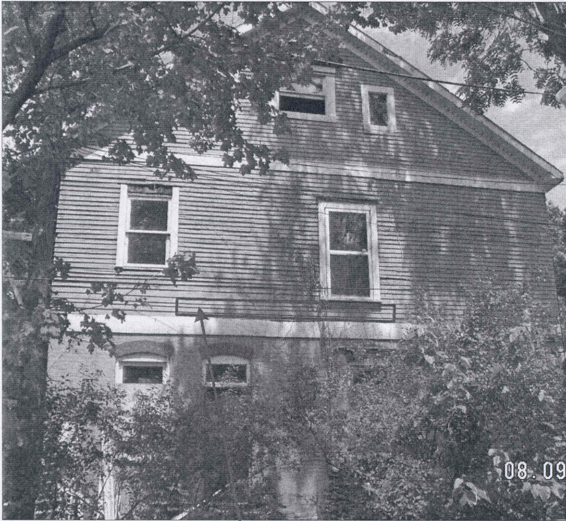
View From South showing Location of Proposed Porte Cochere Attachment to House
