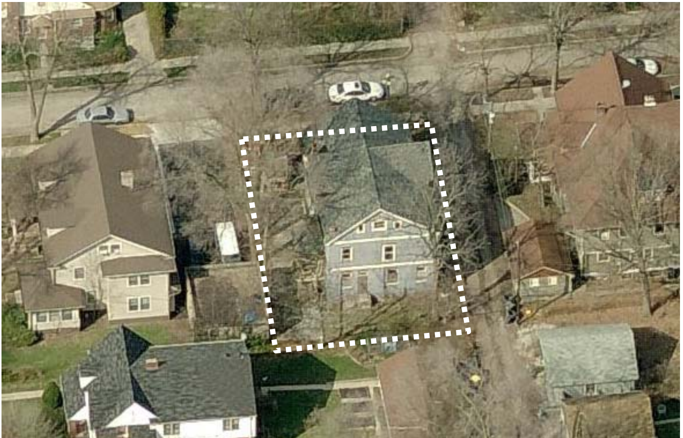
View of the property seen from the south
