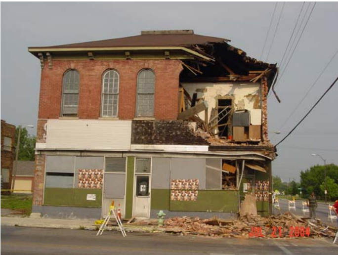
Above: Front elevation after removal of northeast corner.
