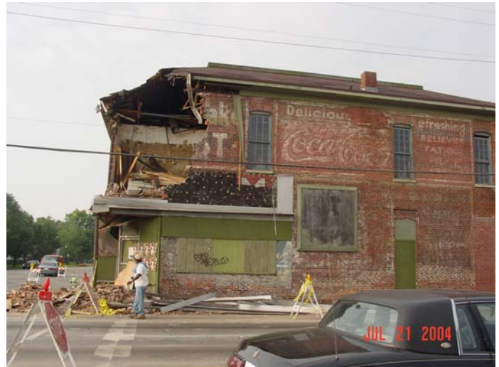
Above: North elevation after removal of northeast corner.
