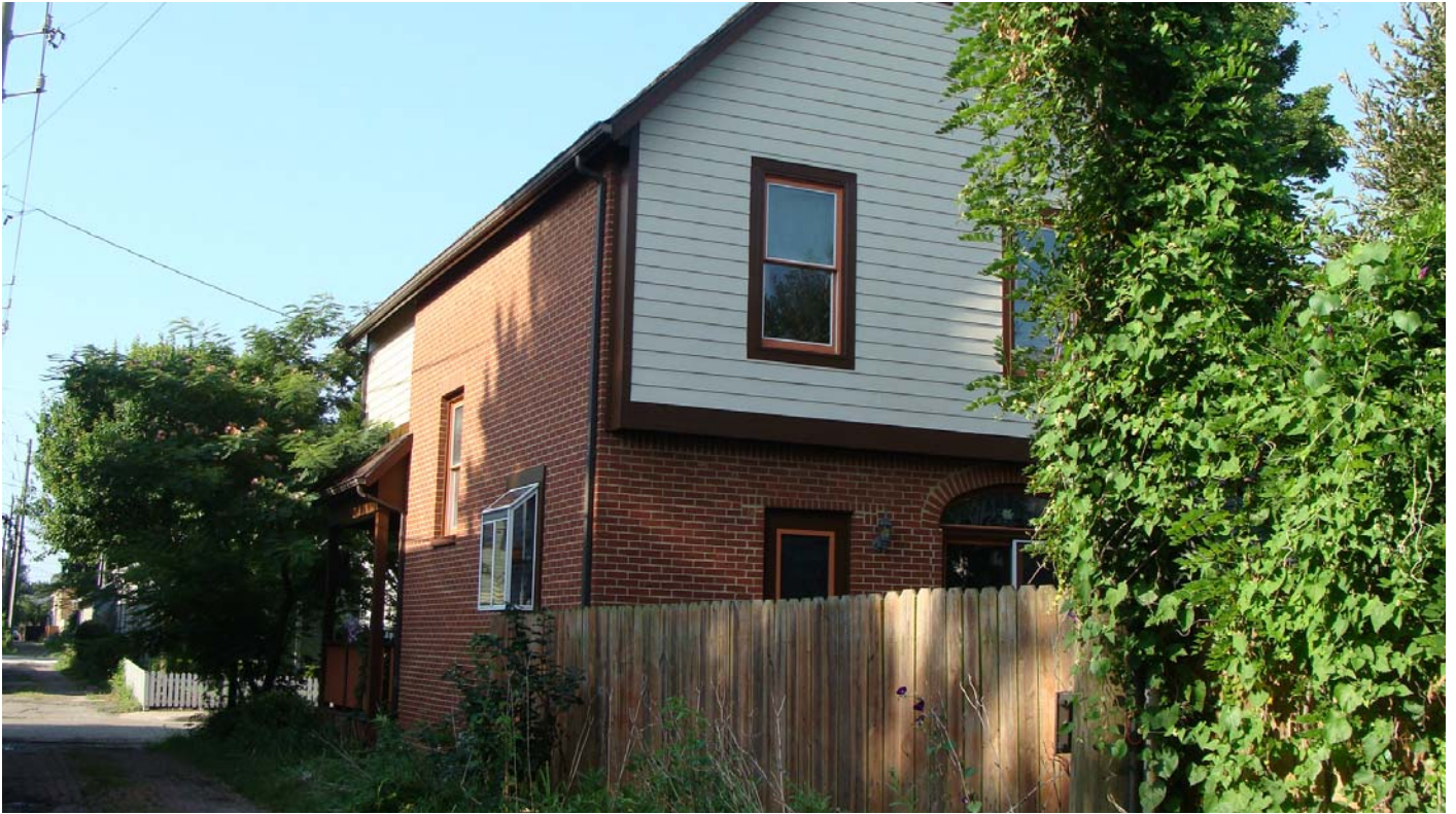
View of back of primary structure seen from the adjacent alley
