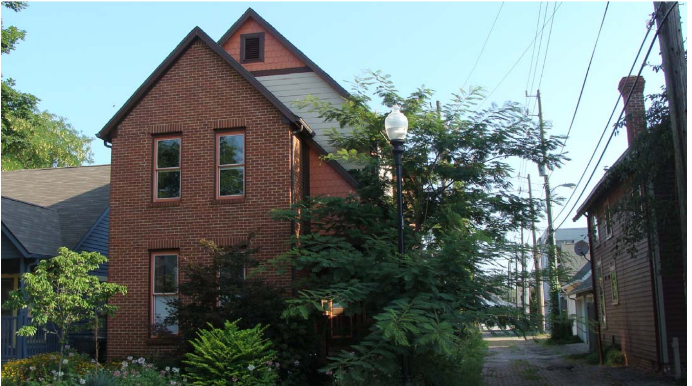
View of front of primary structure
