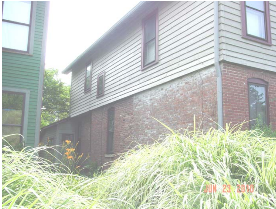
North side elevation from street / rear addition visible
