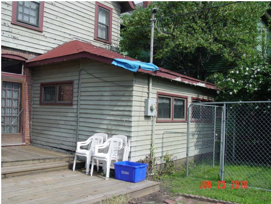
View of rear addition requested to demolish
