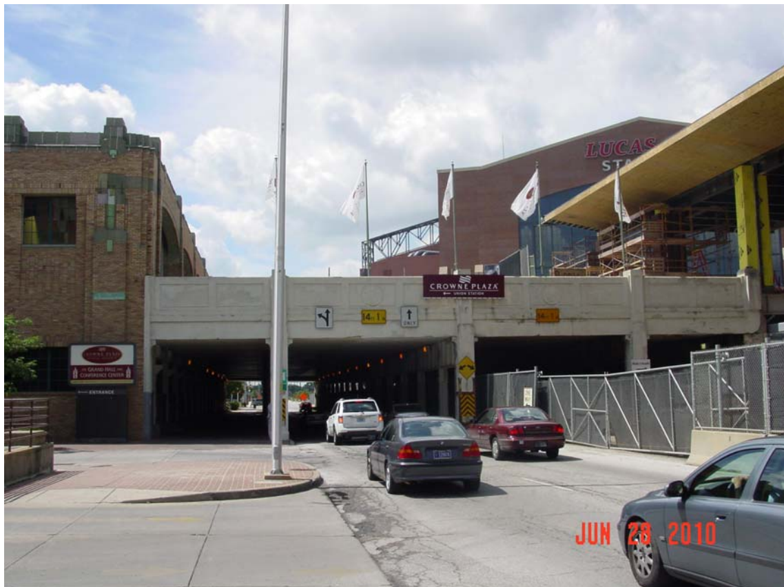
Looking south on Capitol Avenue – View of the bridge on which the pedestrian connector will be built atop.
