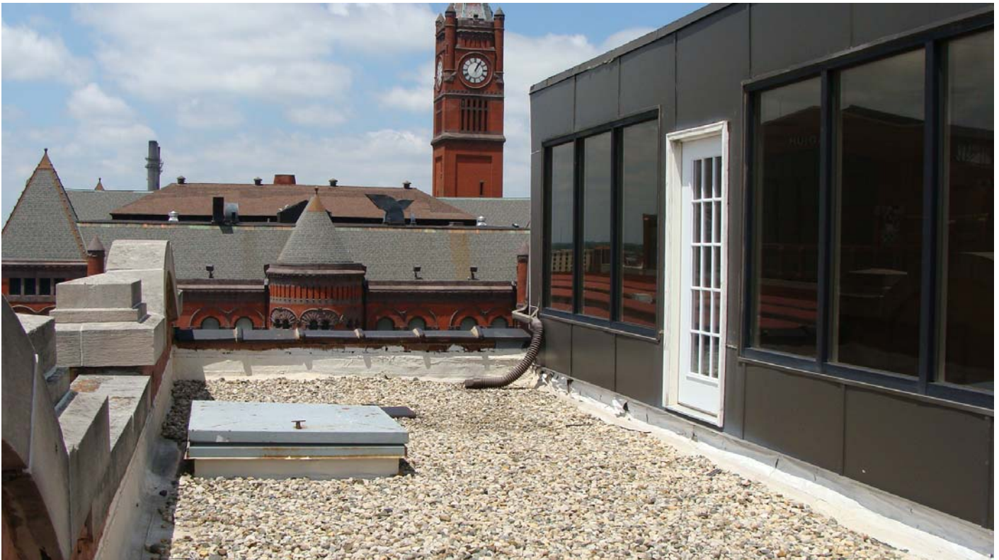
South side of existing penthouse structure as built
