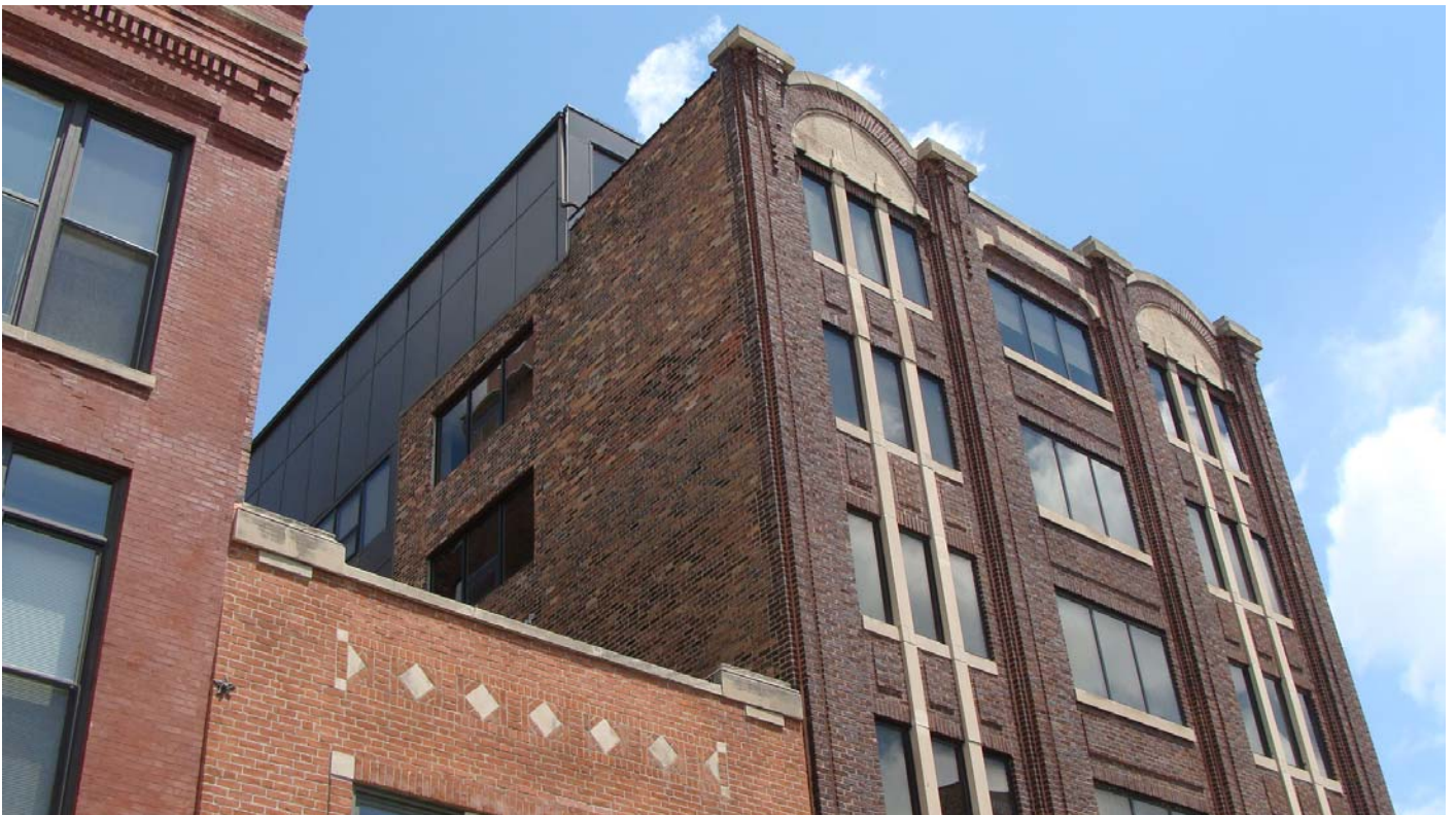
West side of building seen from street level
