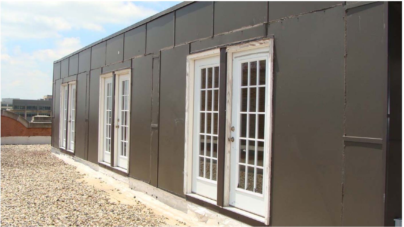
East side of existing penthouse structure as built
