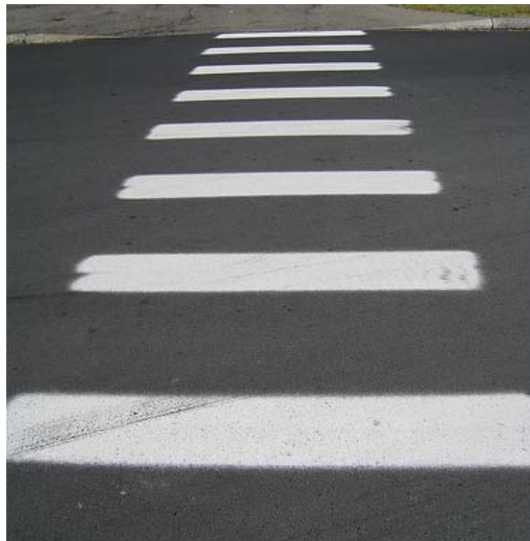
Typical crosswalk lines---to be 24 inches wide
