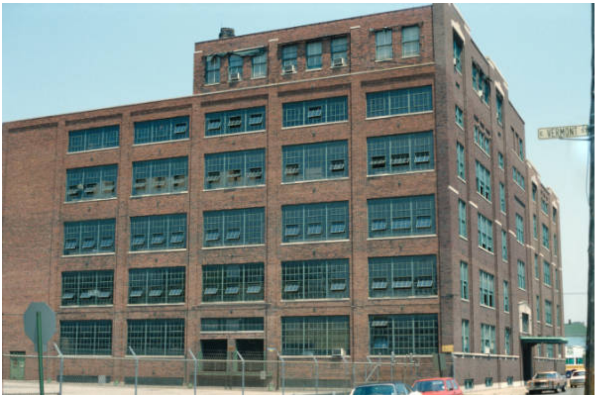
1979 photo showing original steel windows on south side of building
