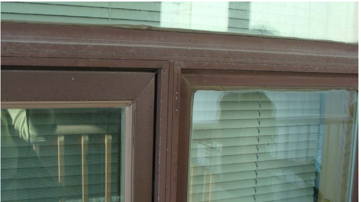
Close up of existing window configuration and detailing
