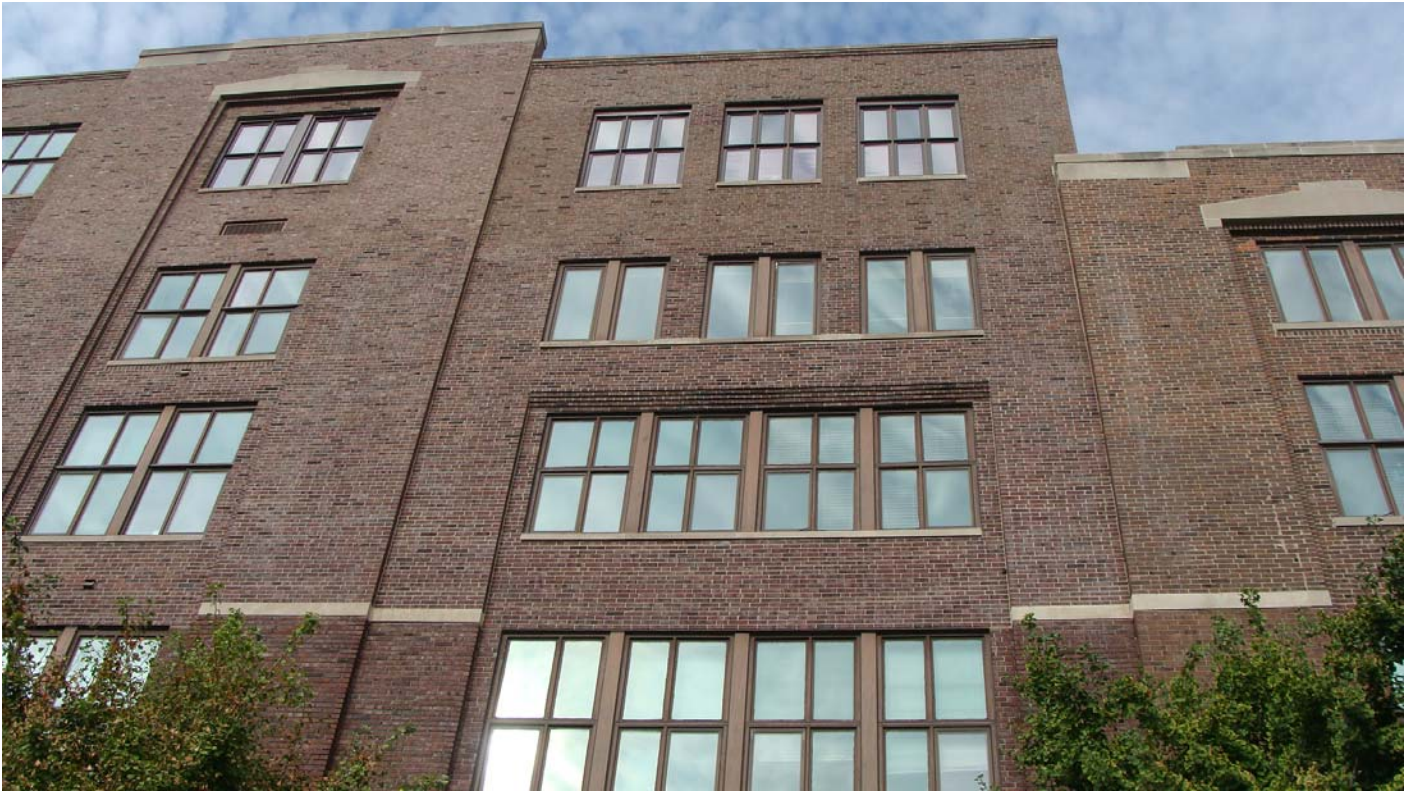
East side of building showing existing windows (Note: top floor windows are new Marvin metal clad units with a 'bronze' finish)
