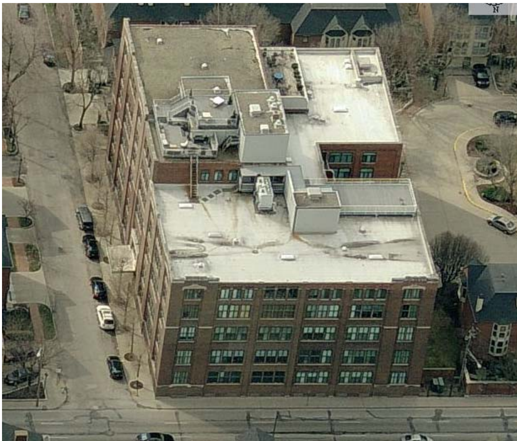
Aerial photo of building looking south
