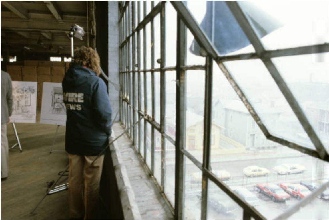
1982 photo showing original steel windows on south side of building
