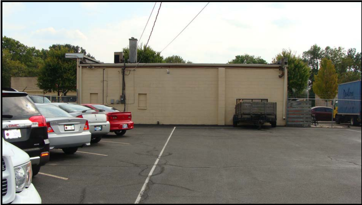
Above: View of back of building
