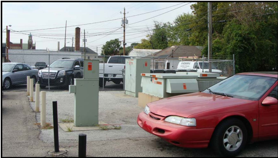
Above: AT and T easement at rear of site
