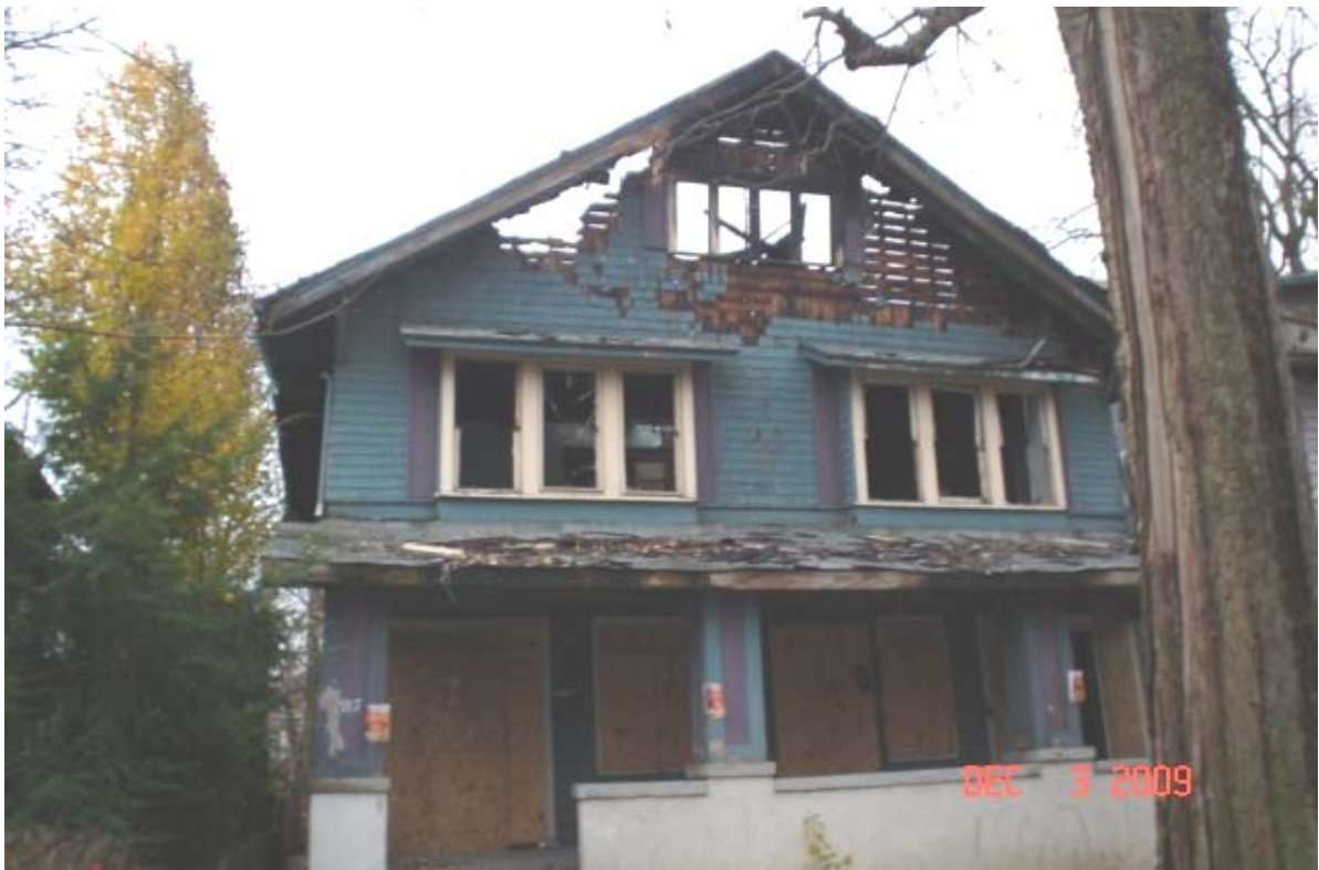
Decemer 2009- front of house before gable was removed by emergency demolition
