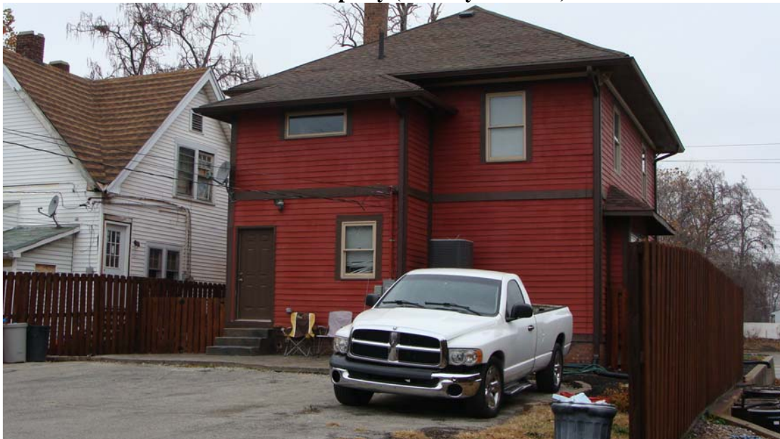
View of East Elevation and Rear Elevation of Structure
