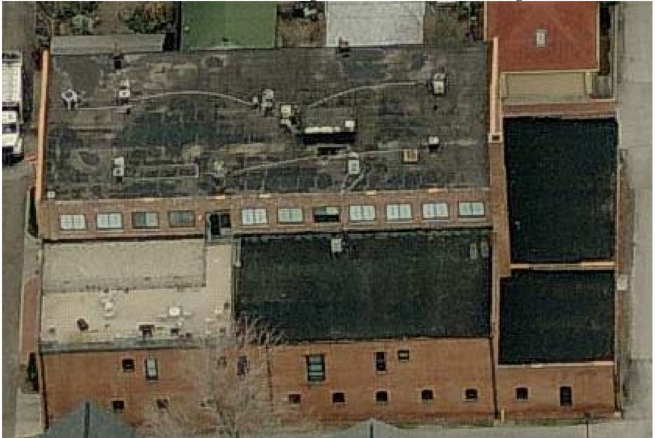
Below: Aerial view looking at south elevation of building.
