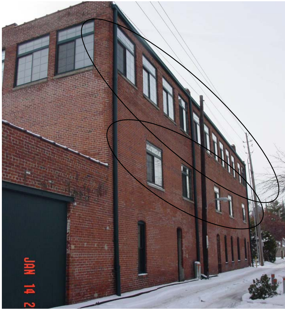
Above: View of the 17 windows replaced on the north elevation
