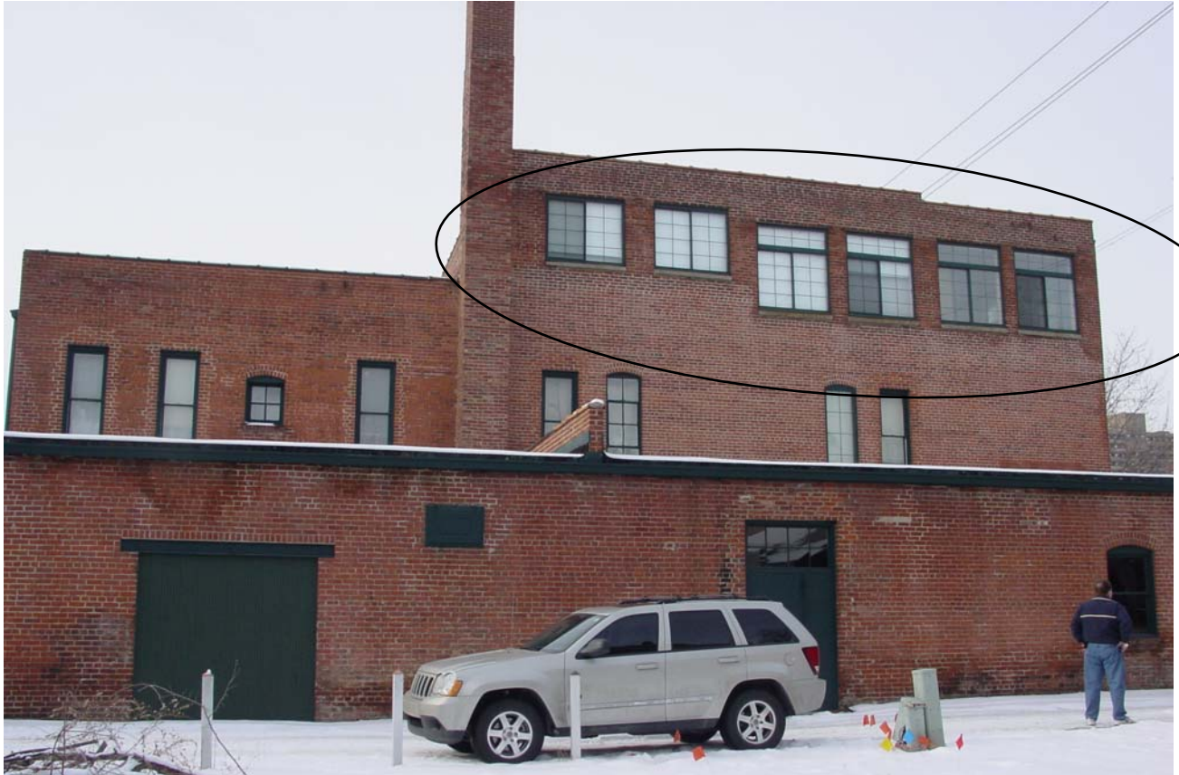
Above: View of the windows replaced on the east elevation
