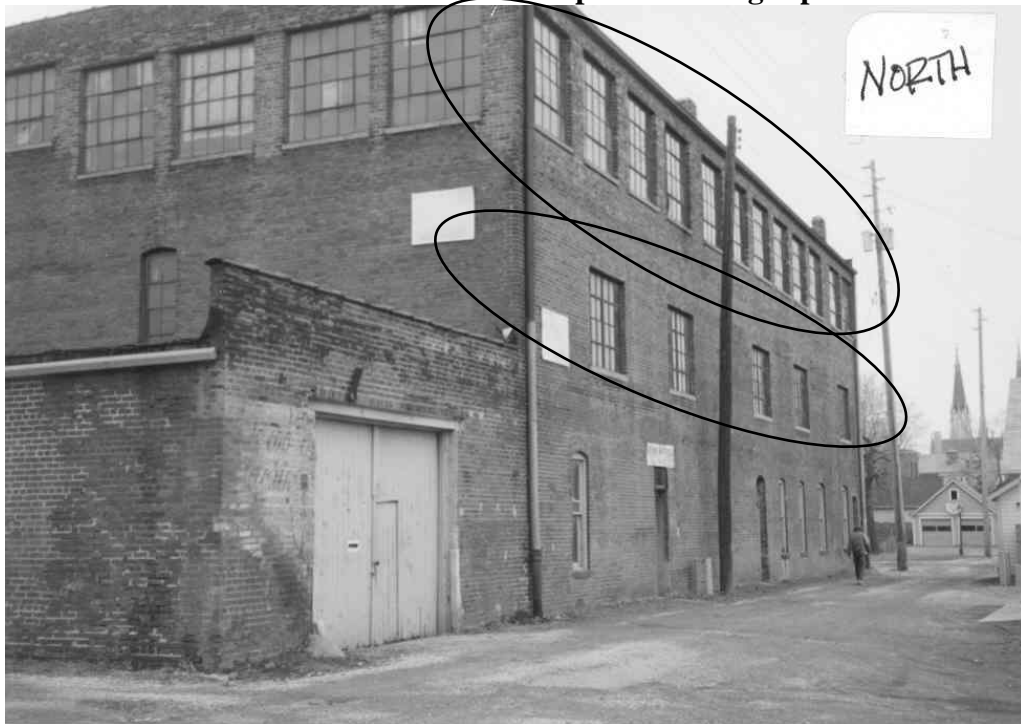
Below: View of the 17 windows prior to being replaced.
