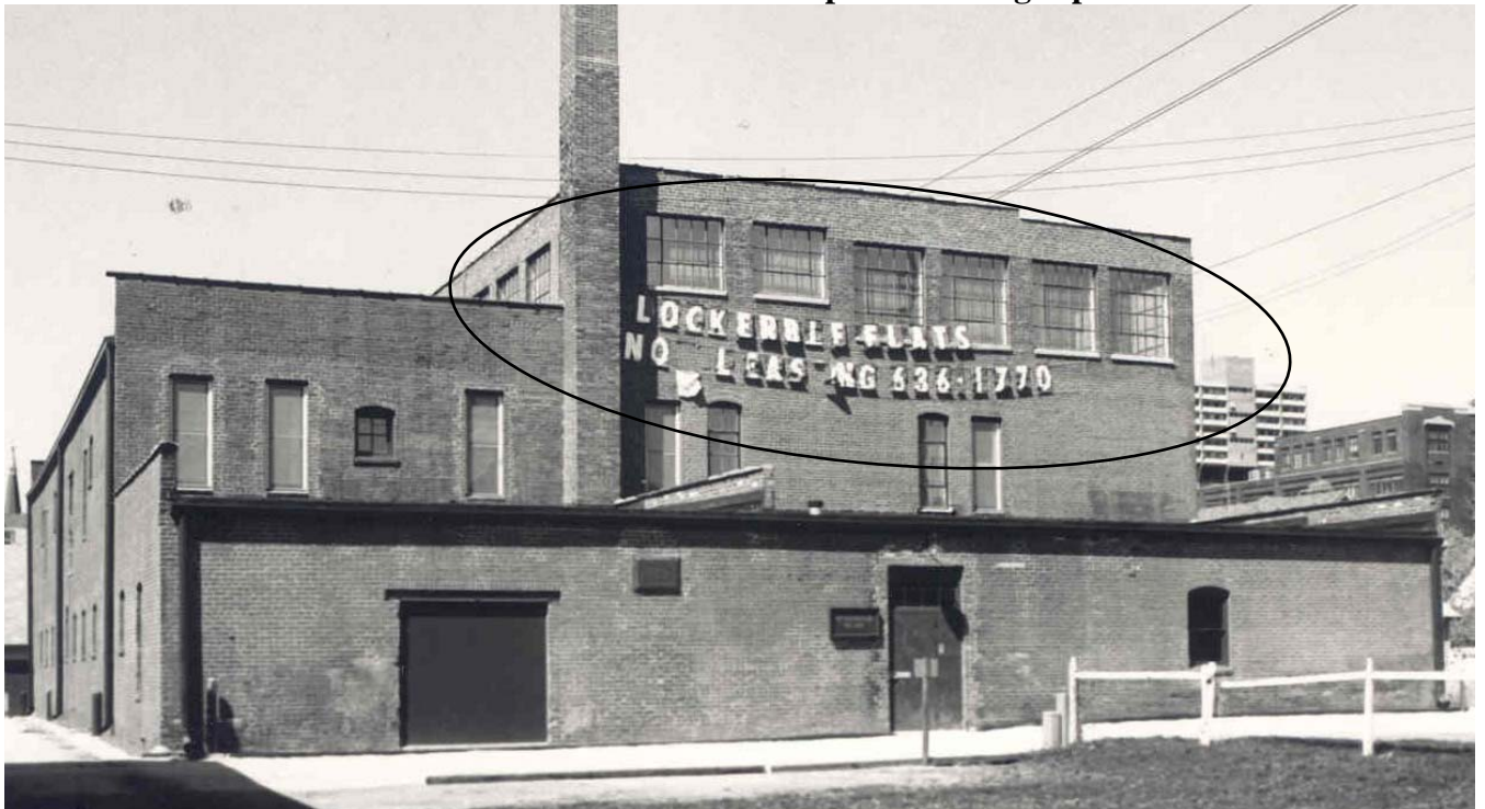
Below: View of the same windows prior to being replaced.
