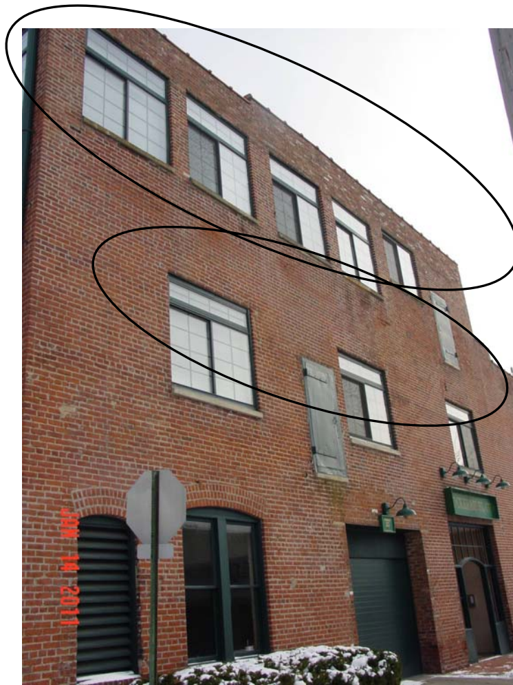
Above: View of windows on the west elevation that were replaced.
