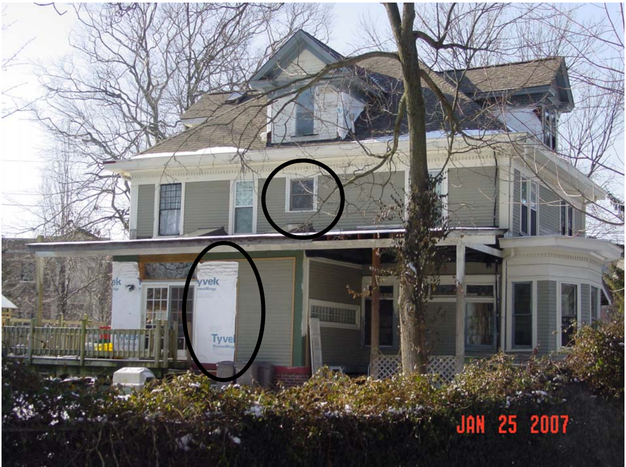
Rear (East) side of House – January 2007
