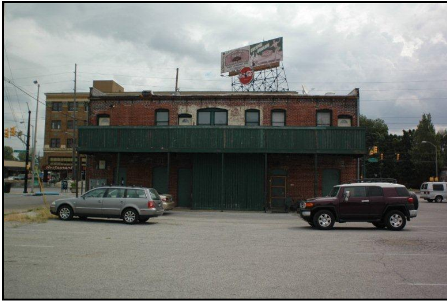
Above: Back of building
