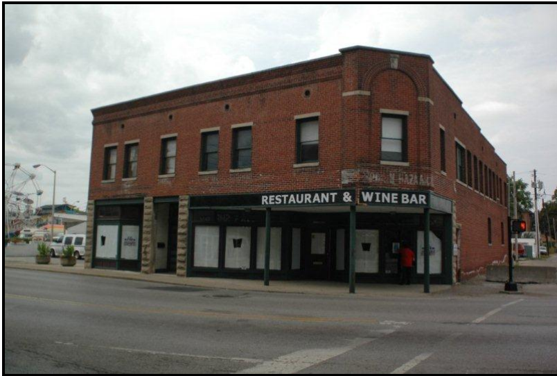
Above: Front of building
