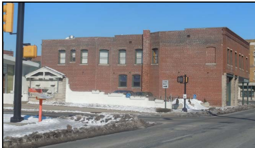
Below: View of south side of the building
