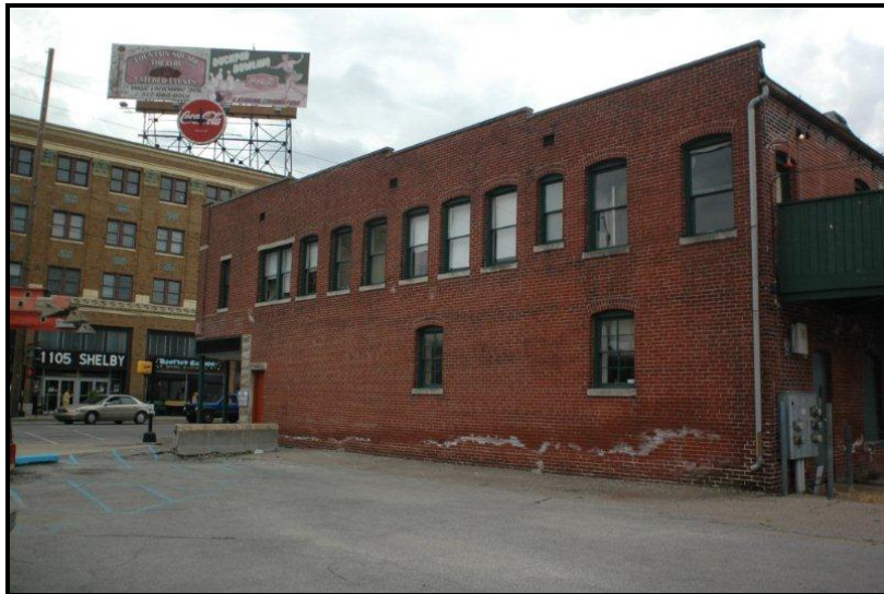
Below: North side of the building
