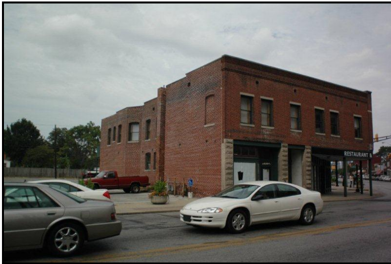
Below: Front and south side of the building
