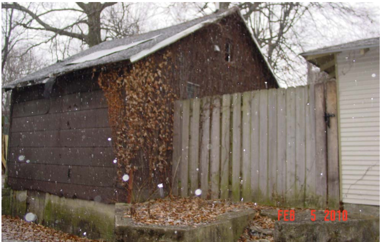
East side of historic garage taken from the alley (Note: original garage door filled in)
