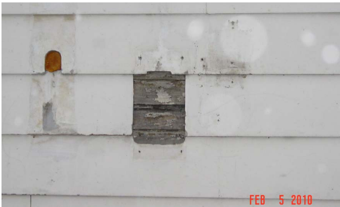
Existing metal siding on historic garage with original wood siding below
