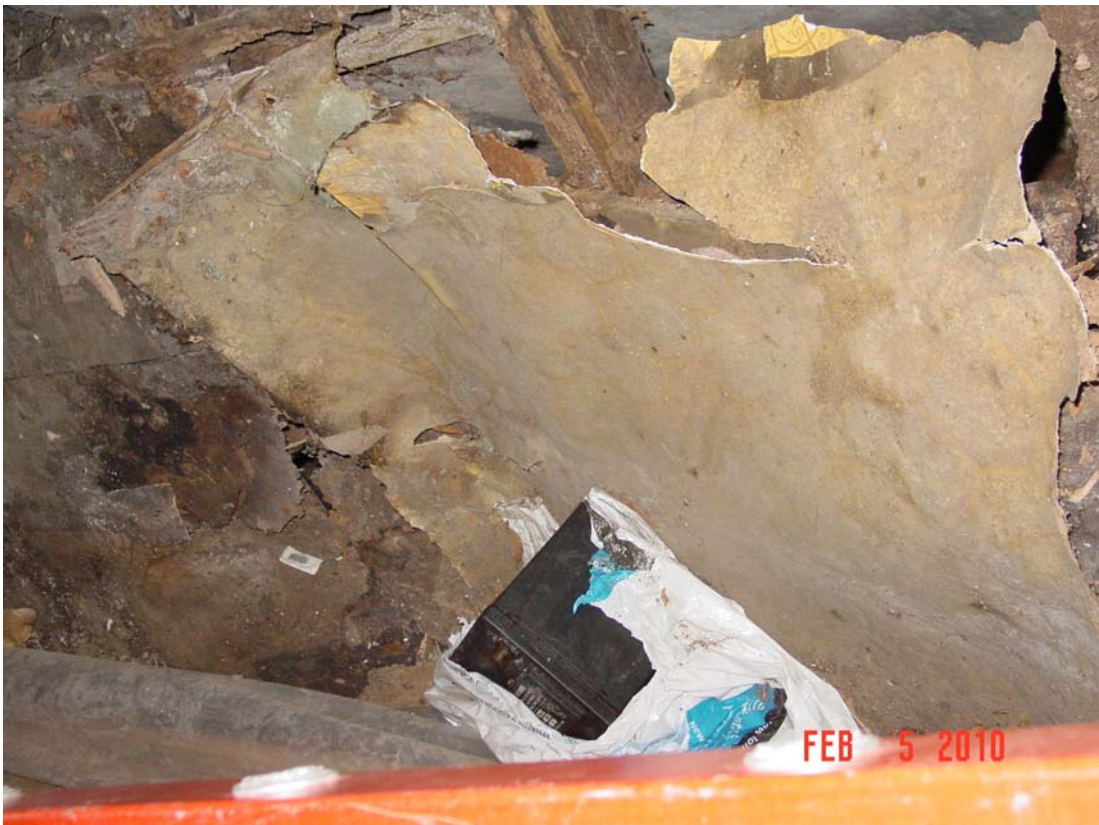
Interior condition of exterior walls
