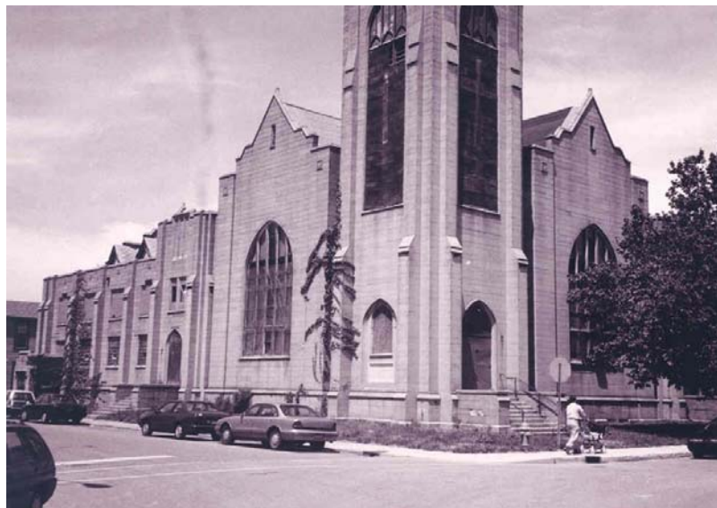
Looking northwest at former church
