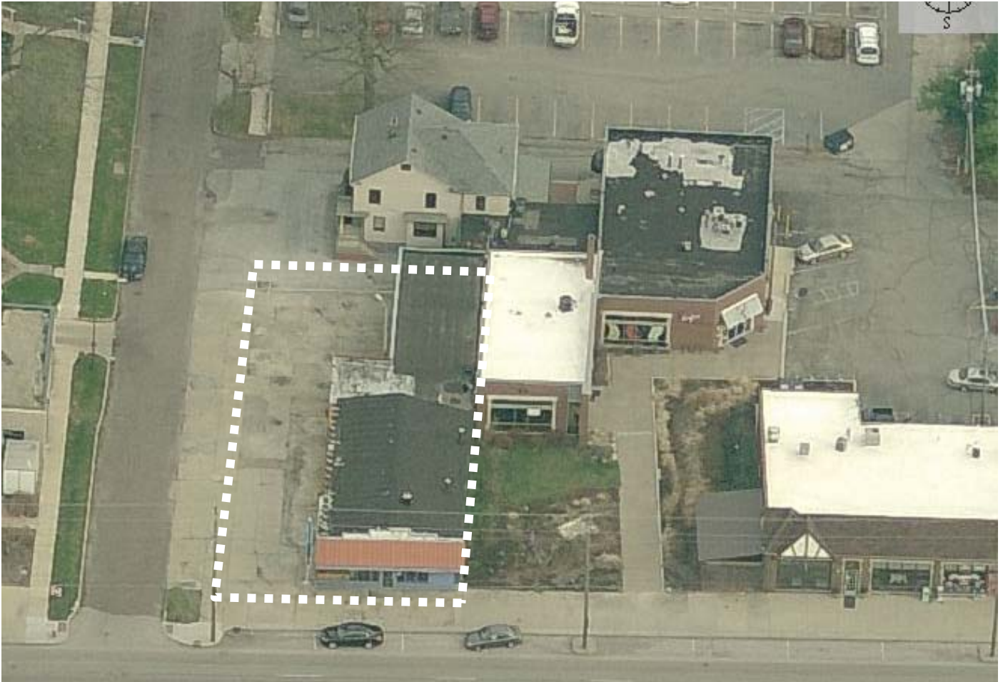
Aerial Photo looking toward front of building
