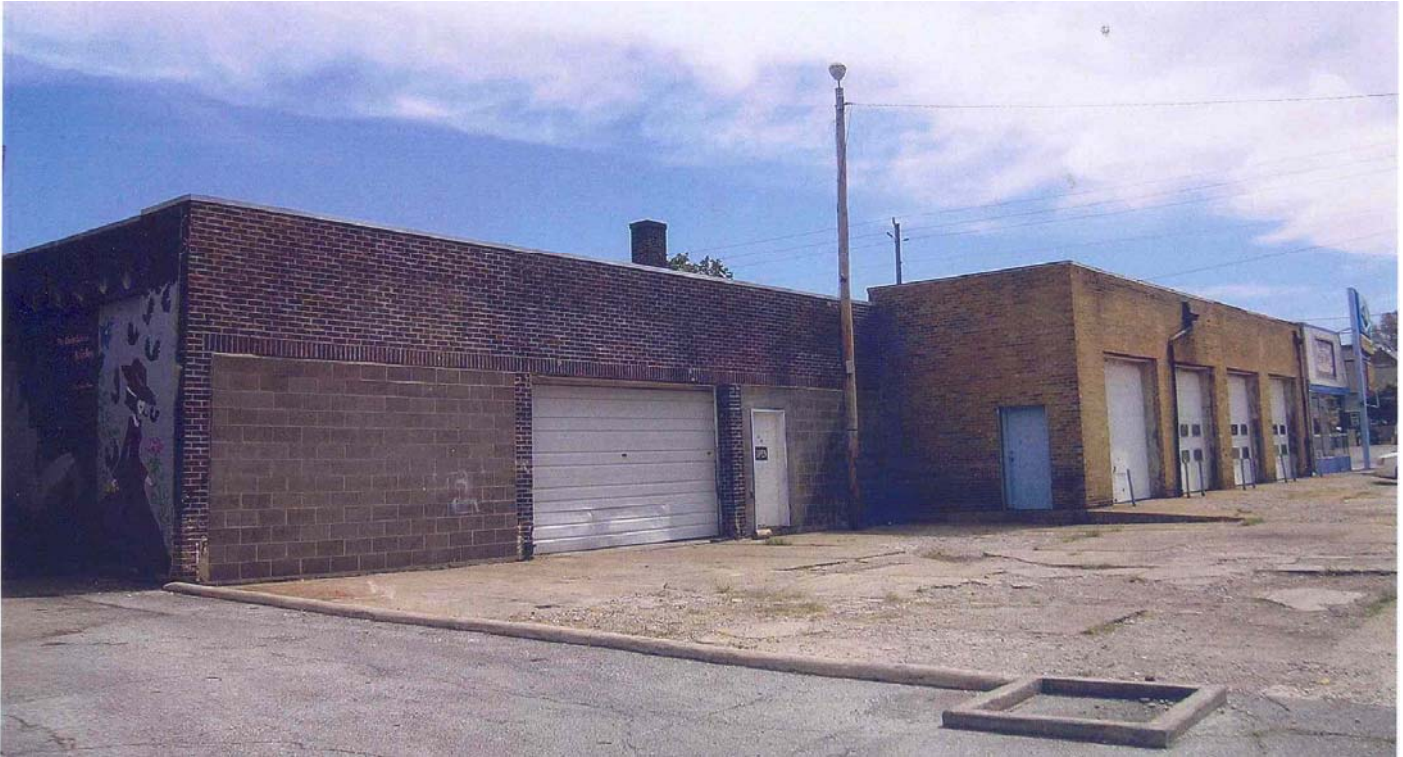
West side of building seen from Layman Street (looking southeast)
