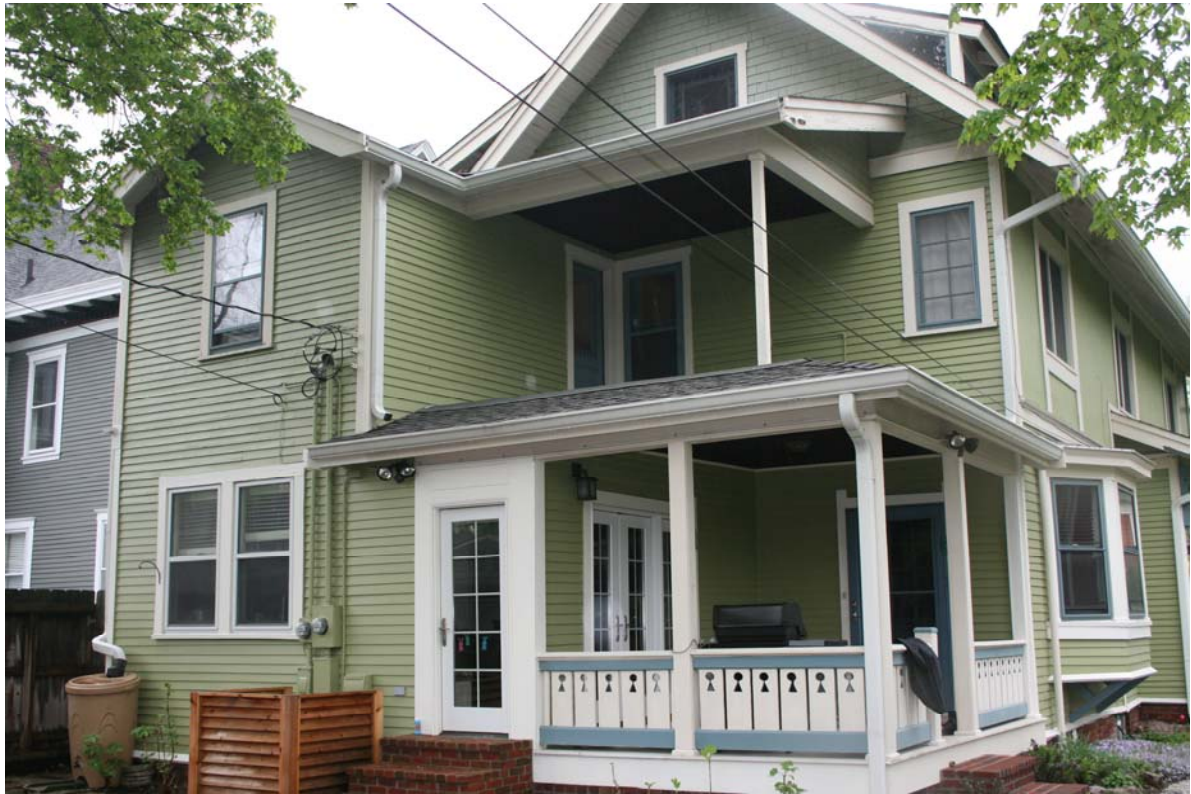
Existing conditions at rear of house
