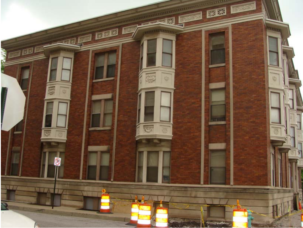
Above: View of south elevation Below: View of courtyard (south)
