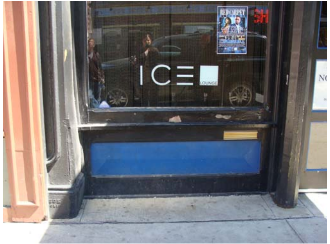
Above: Bulkhead Panels at 235 S Meridian
