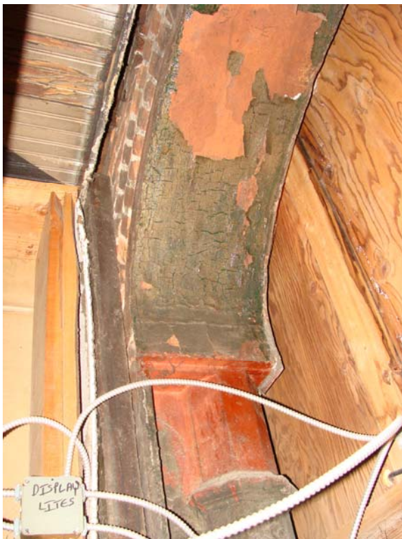
Below: Existing Cast Iron beneath storefront
