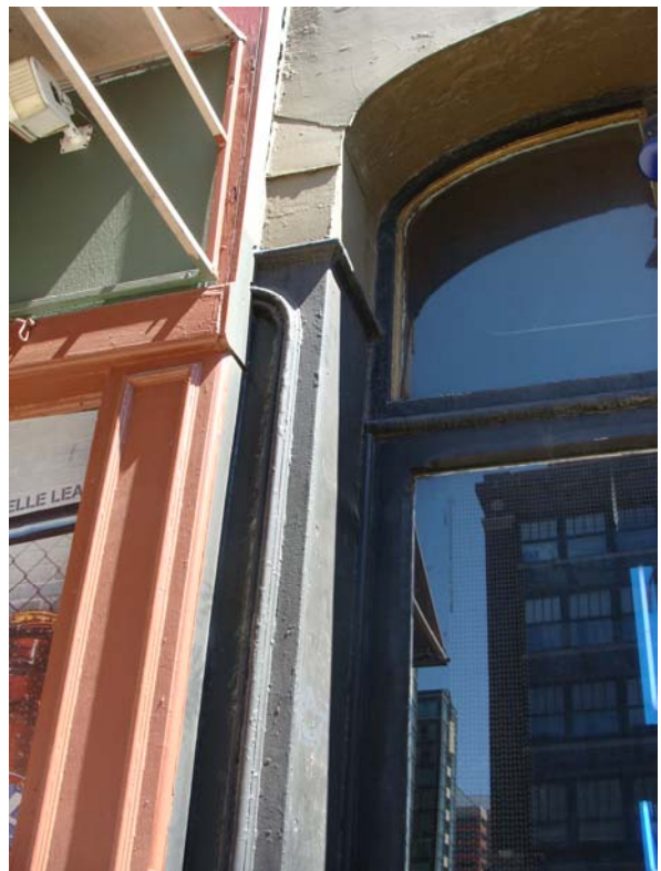
Below: View of wood storefront over iron.
