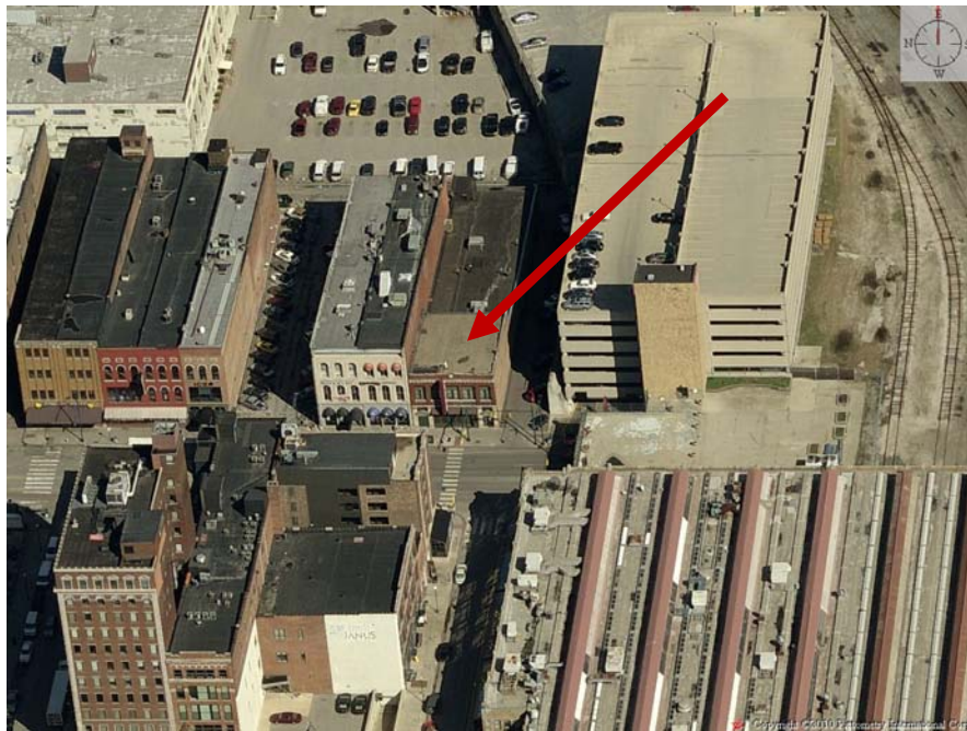
Aerial view looking east
