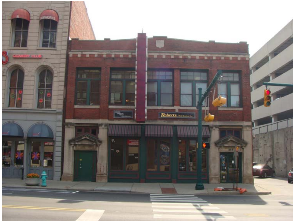
Front Façade - current
