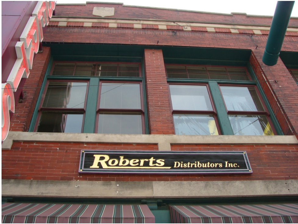
Double-hung sash and transoms on second story
