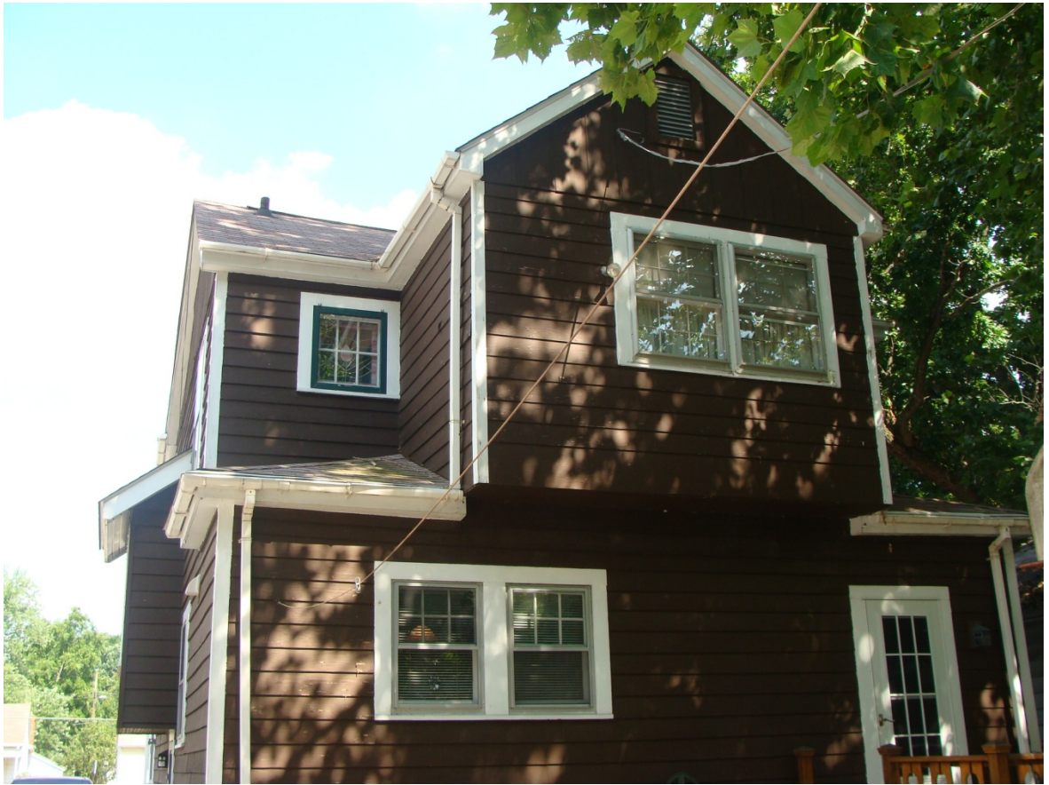
View of rear (west) façade
