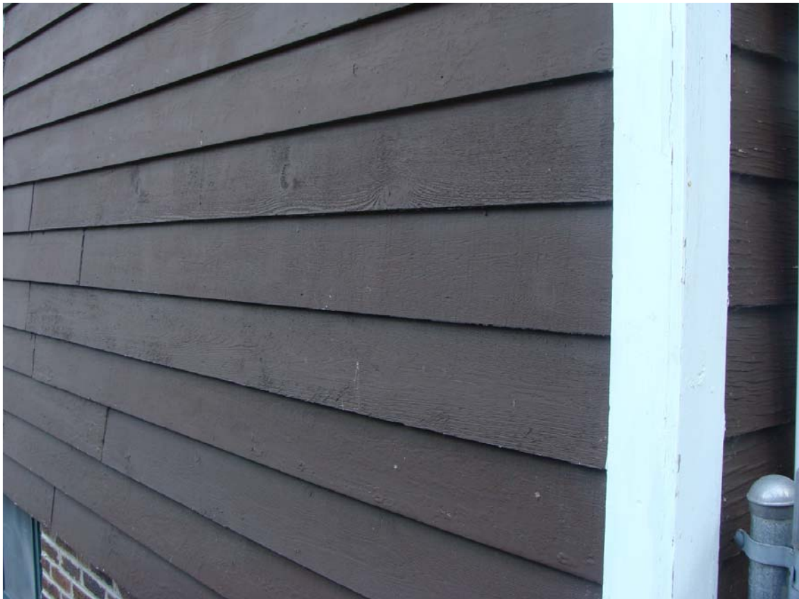
Existing rough finish cedar siding
