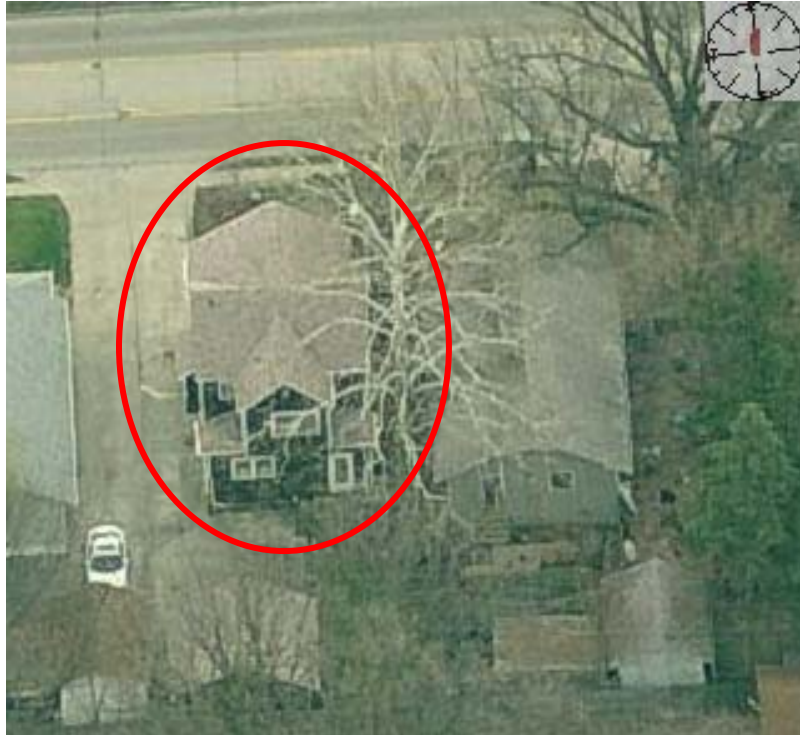
Aerial view of property looking east towards rear (west) façade
