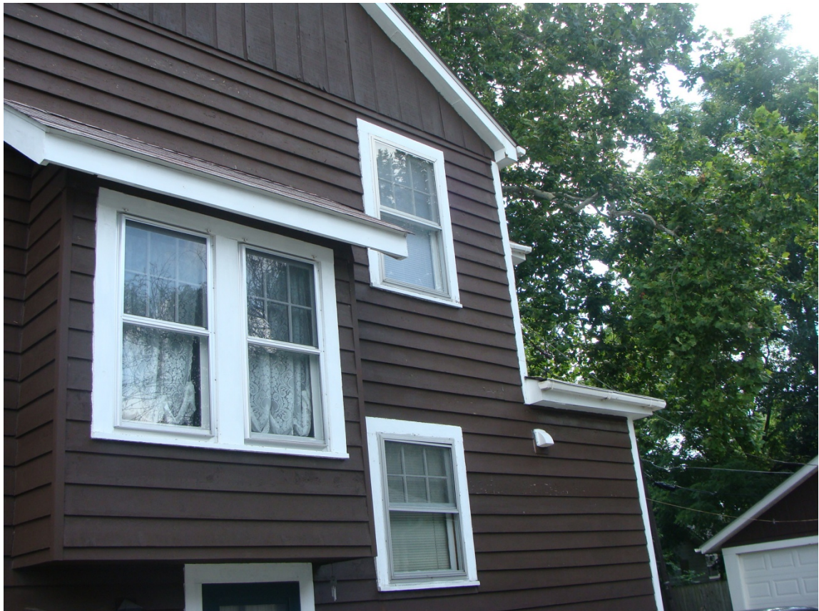
View of north façade
