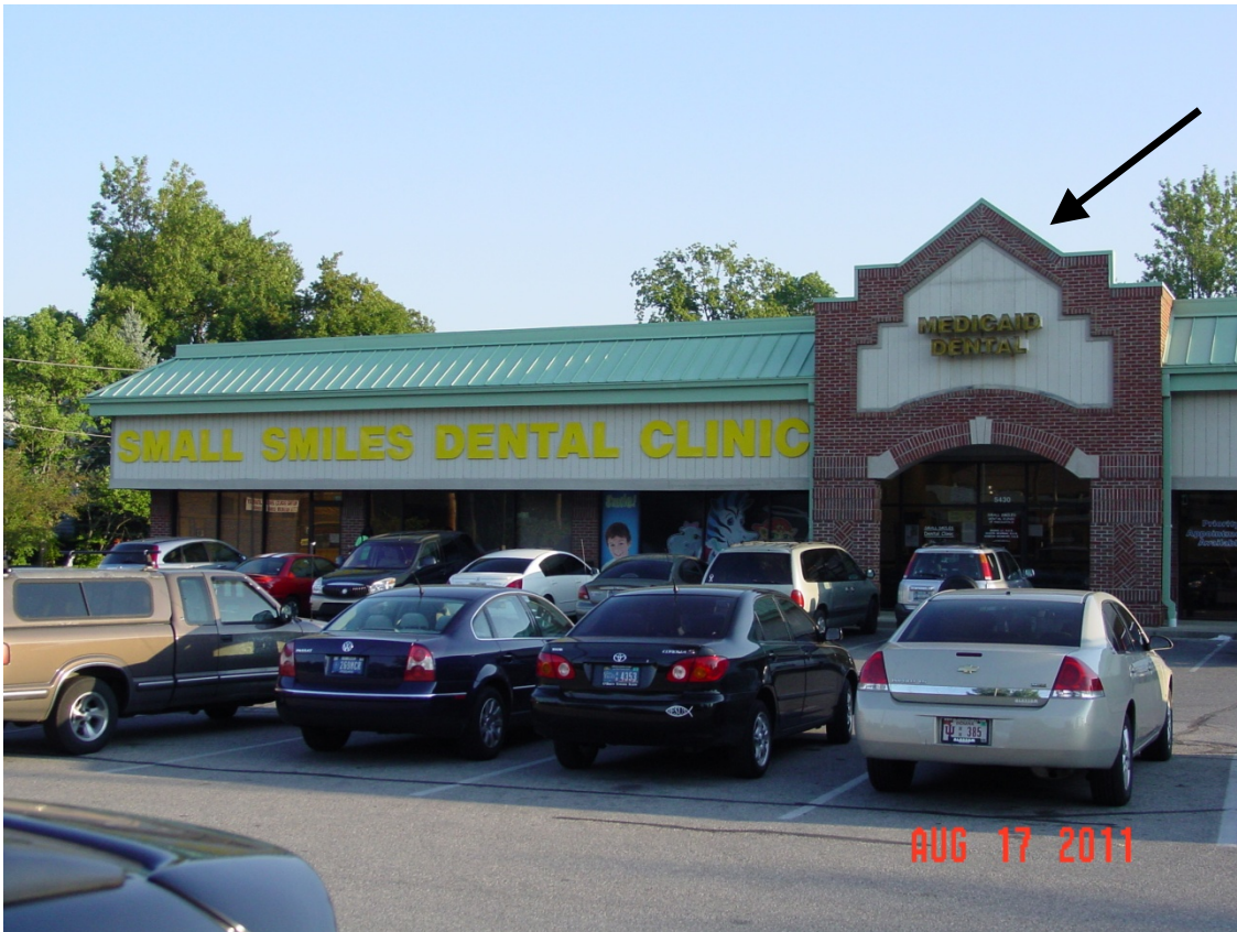
Applicant's storefront with proposed sign location indicated by arrow
