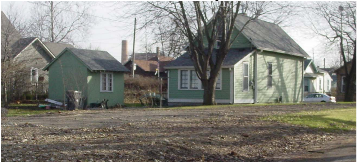
Above: Rear of Cottage
