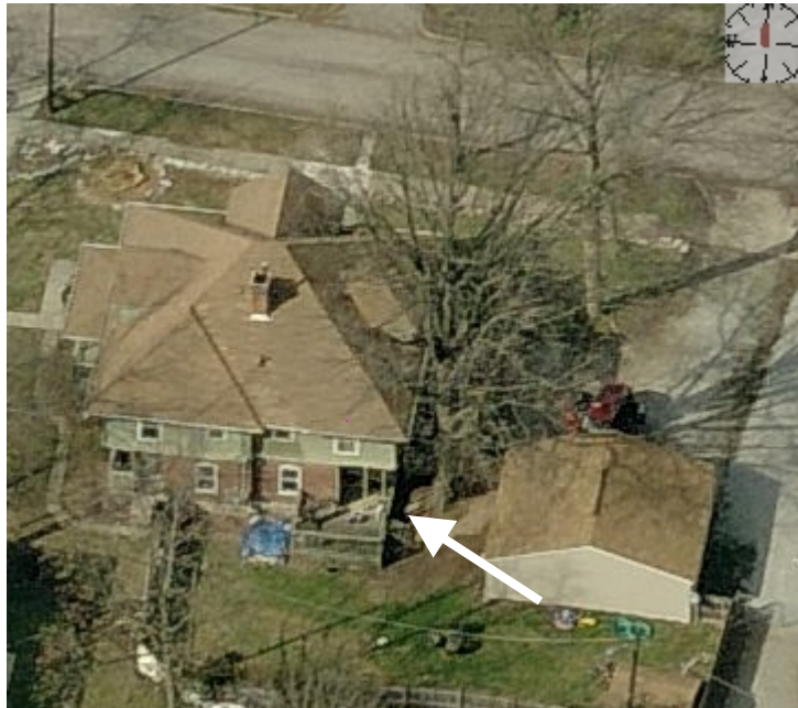
Aerial view of property looking north towards rear (south) façade, with project area indicated by arrow
