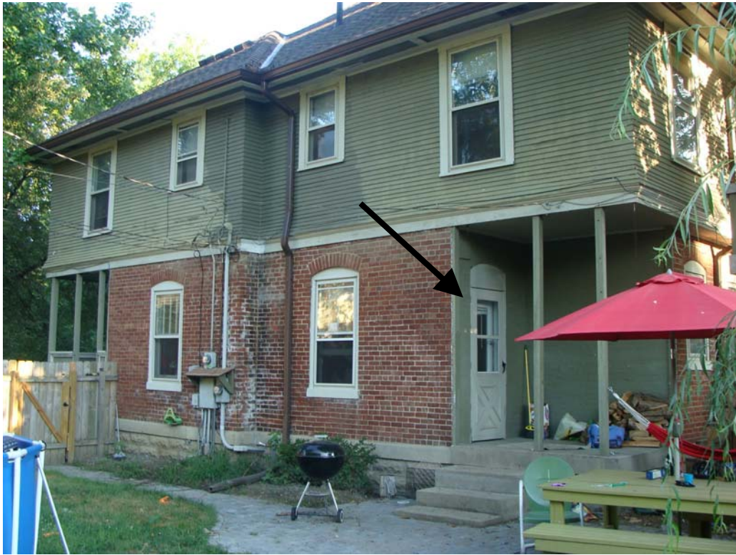
View of rear (south) façade with project area indicated
