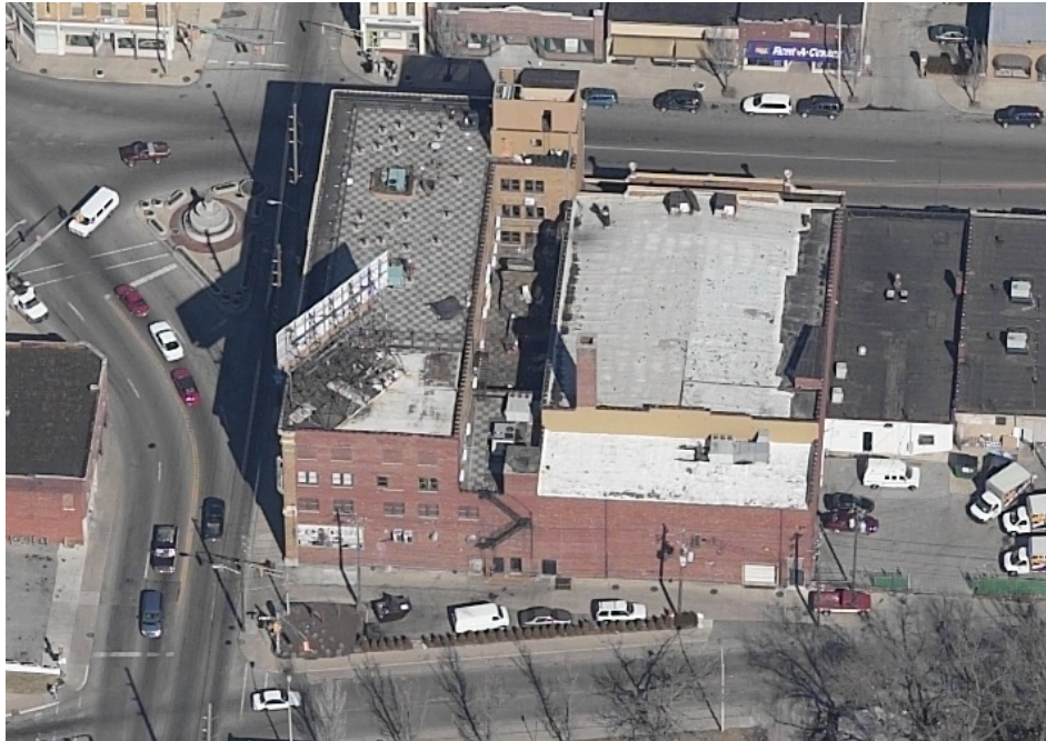
Above: View of building
