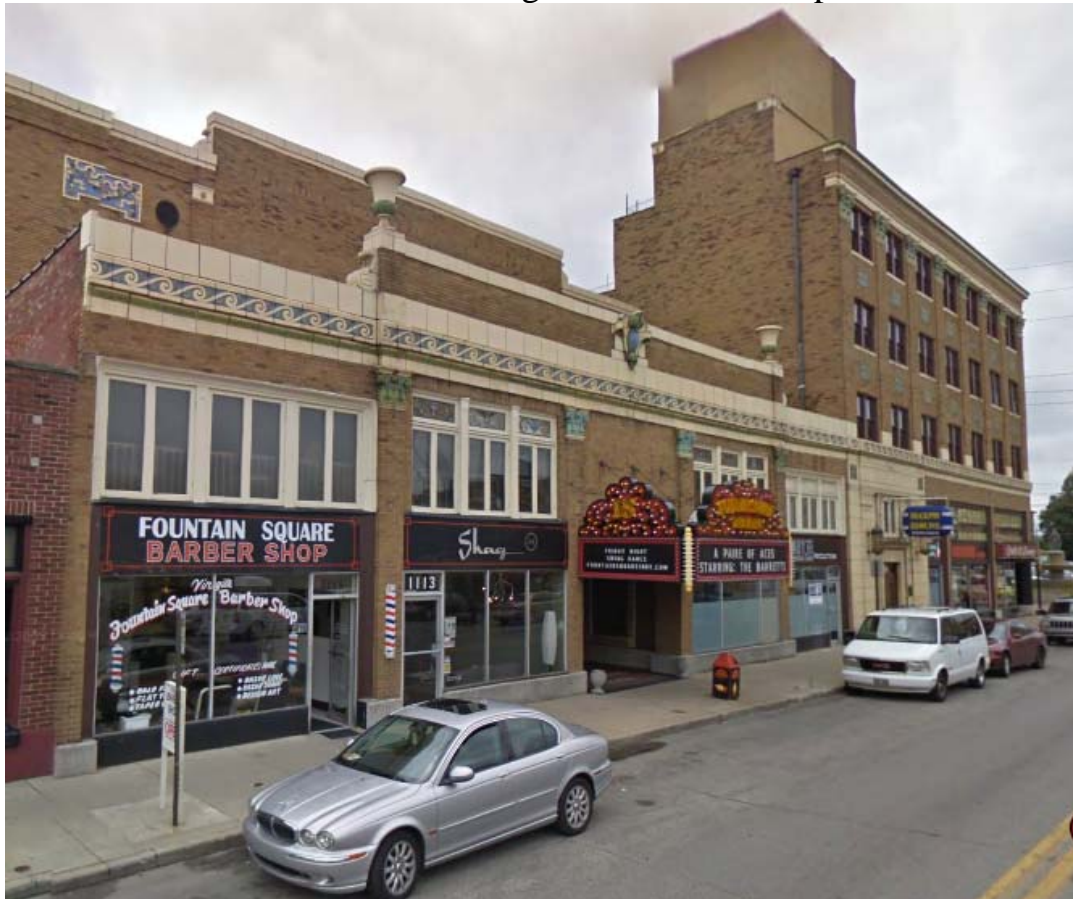
Below: View of building as seen from Prospect St.
