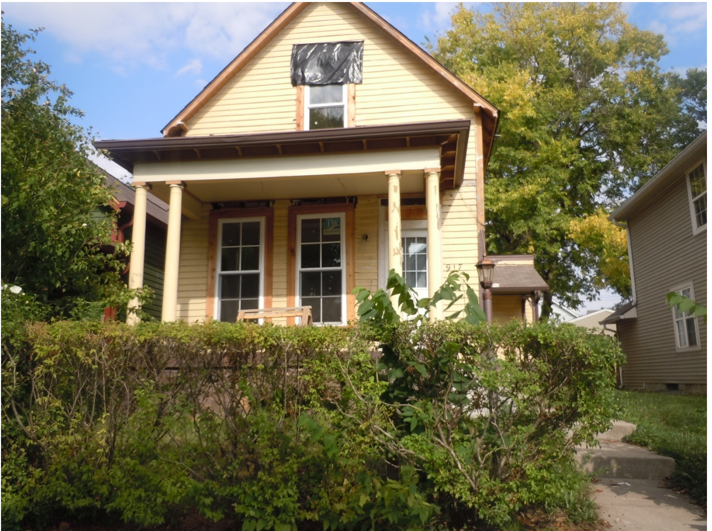
View of property – front (west) façade
