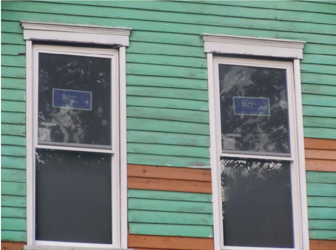
Above: View of porch railing installed Below: View of extruded vinyl windows installed at second floor front elevation.
