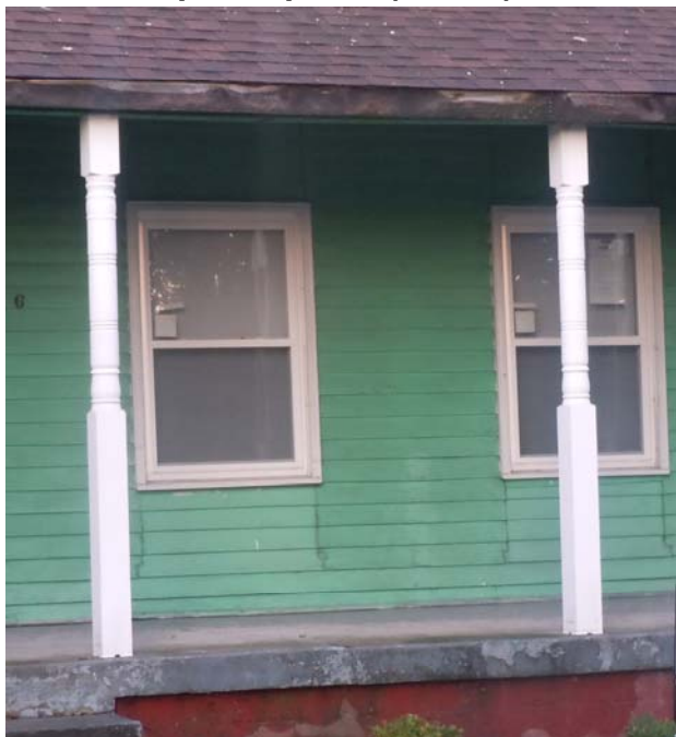
Above: Outline of original length of window seen in siding Below: View of new porch posts (on left) View of typical porch post in Cottage Home
