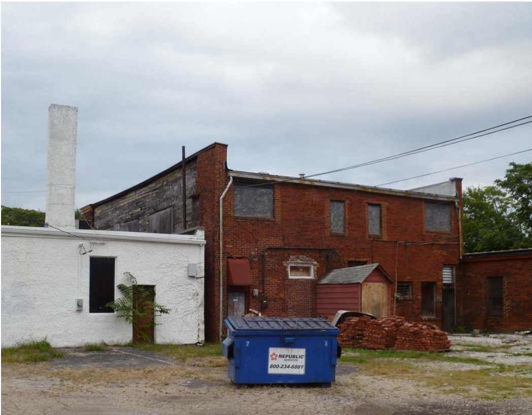
View of rear façade & north wall from alley
