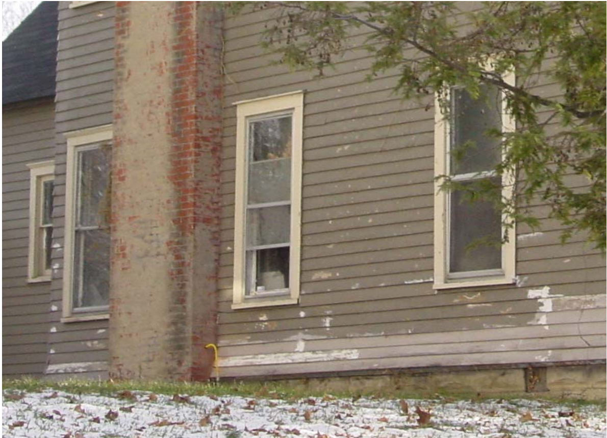
Above: View of wood windows covered by aluminum storms on north elevation before replacement. Below: View of aluminum clad windows installed and new wood trim installed.
