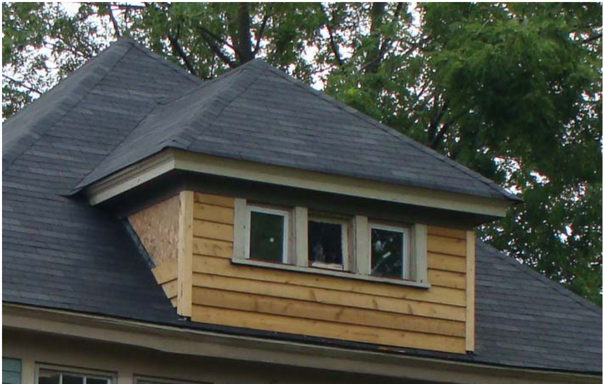
Above: View of original wood shingles in dormer Below: View of wood lap siding used to replace shingles
