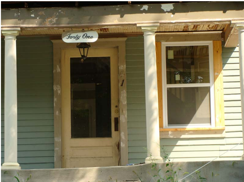
Above: View of original window and trim at front porch window Below: View of new vinyl window and wood trim. Window is shorter and wider than the original.
