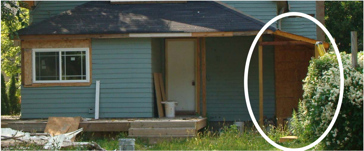
Above: View of shed-like structure as it appears today
