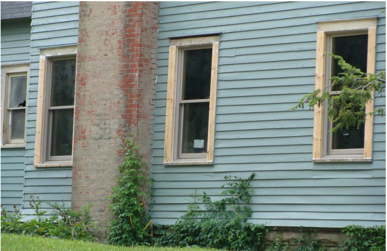
Above: View of wood windows covered by aluminum storms on north elevation before replacement. Below: View of aluminum clad windows installed and new wood trim installed.
