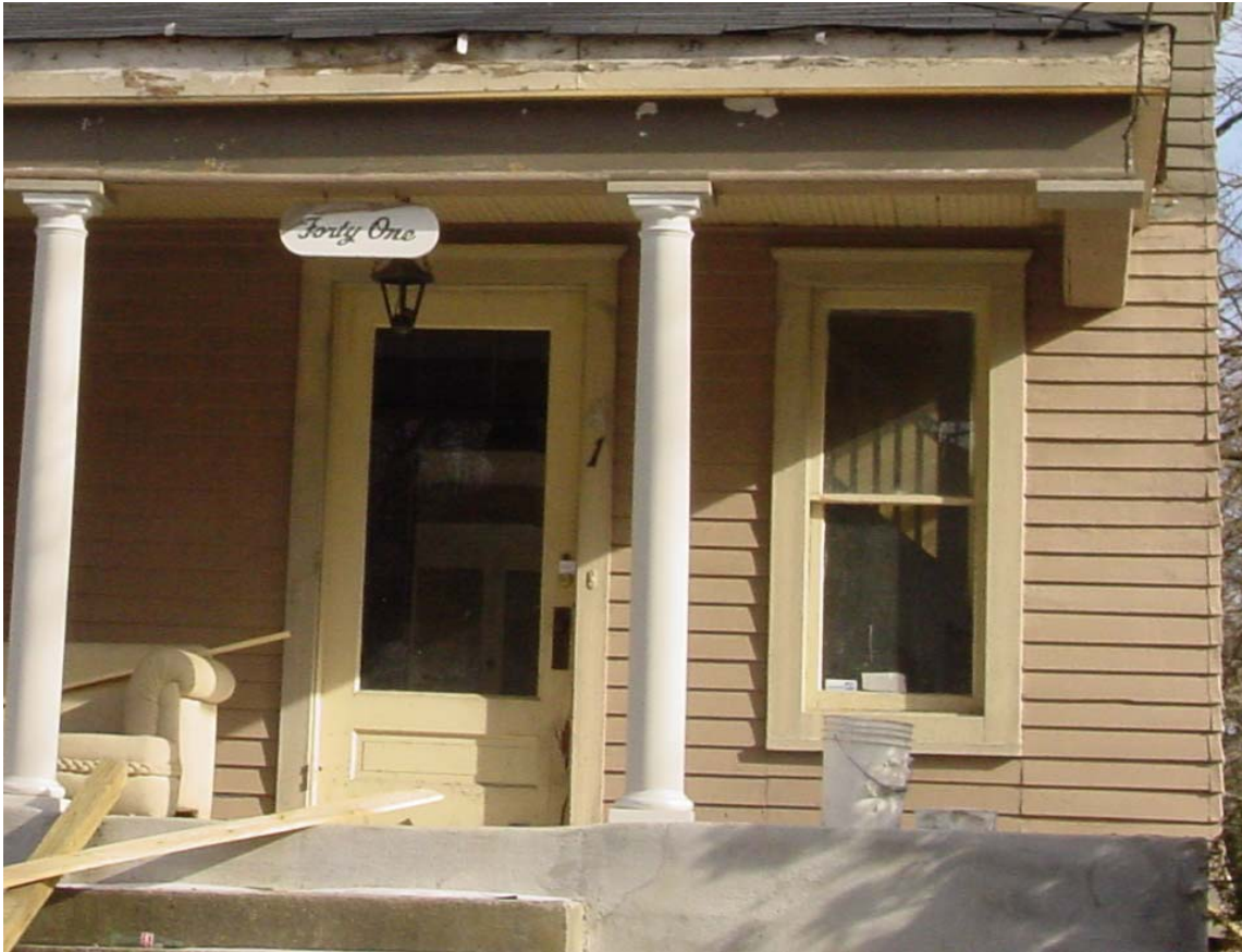
Above: View of original window and trim at front porch window Below: View of new vinyl window and wood trim. Window is shorter and wider than the original.
