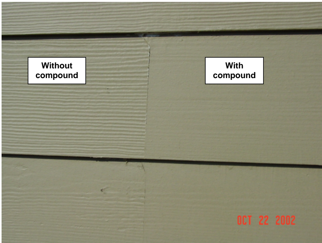
View of siding with and without Elastomeric Patching Compound on similar property in St. Joseph Historic District approved in November 2002
