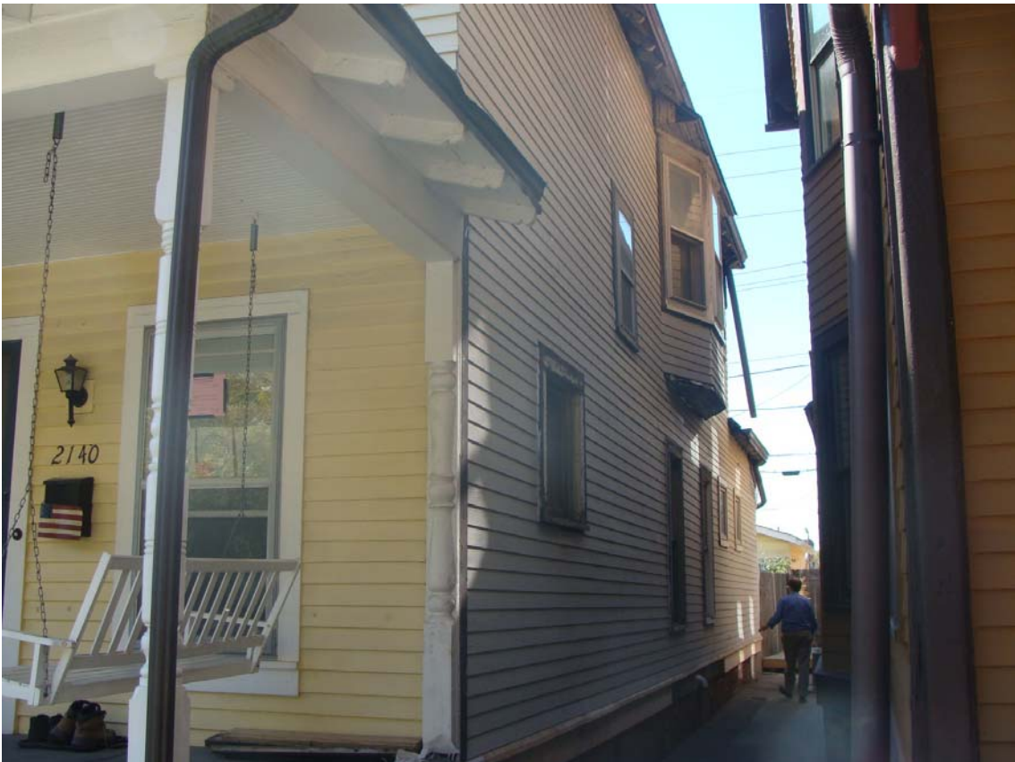
View of north façade with siding work completed
