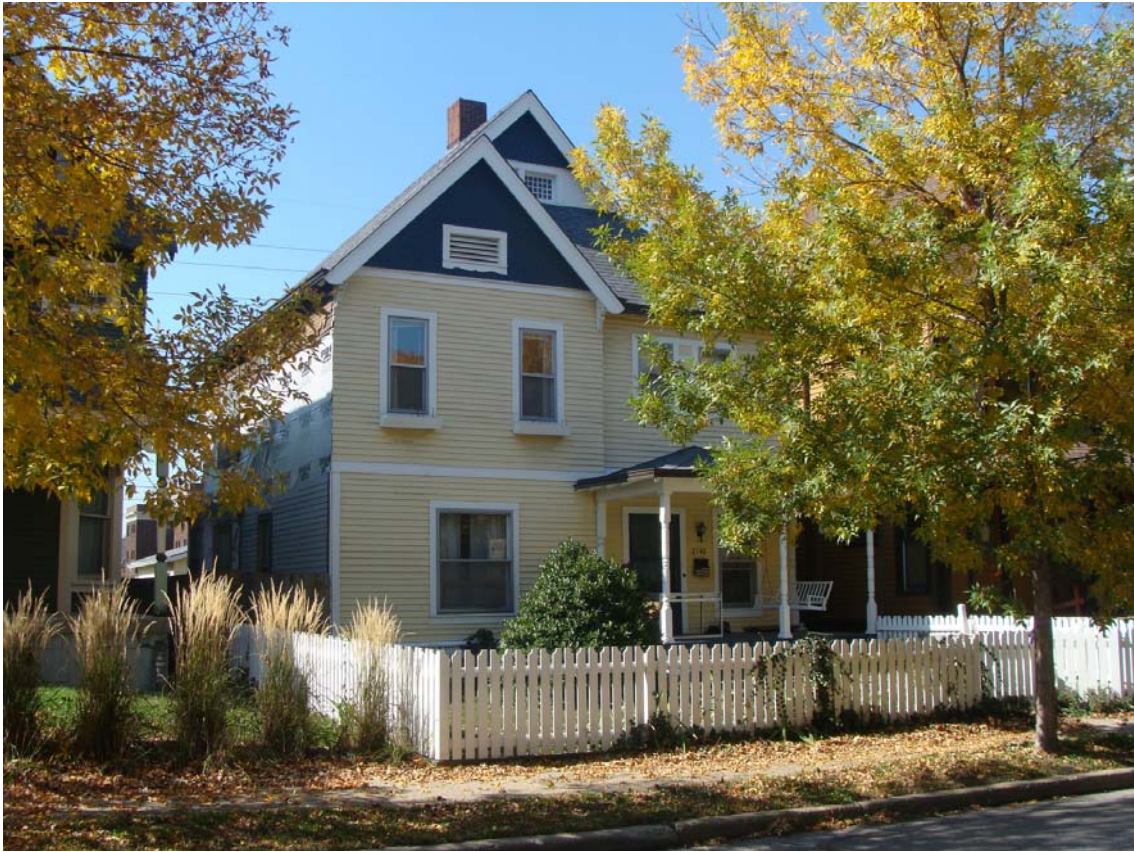
2140 N. Pennsylvania, partially completed siding work visible on the south façade
