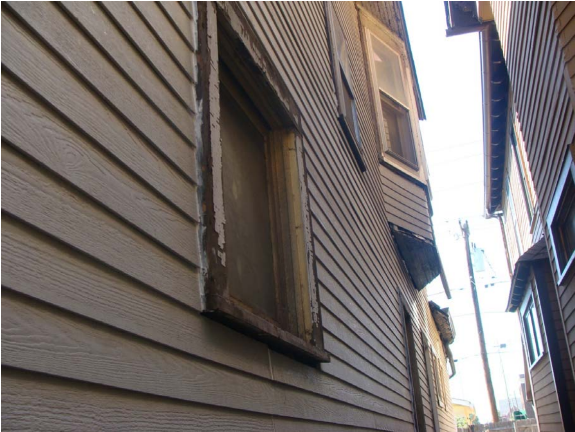
View of siding texture – north façade
