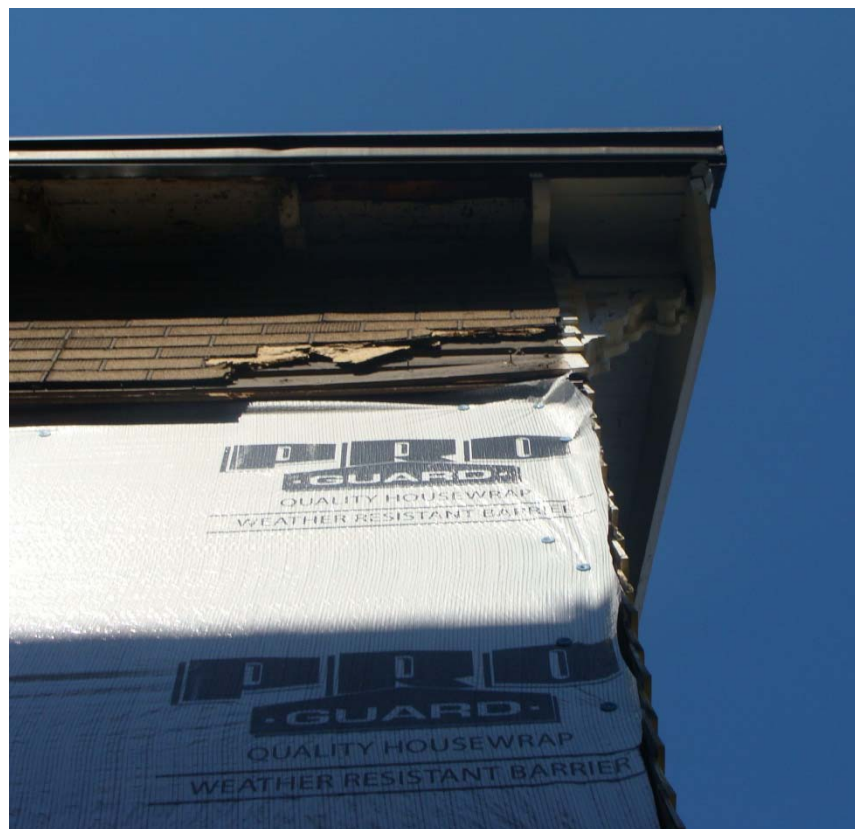
Insulbrick and original wood siding visible on south façade
