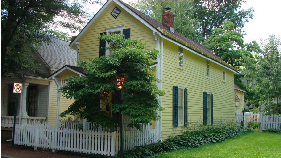
Federal-style house at south end of Park Avenue
