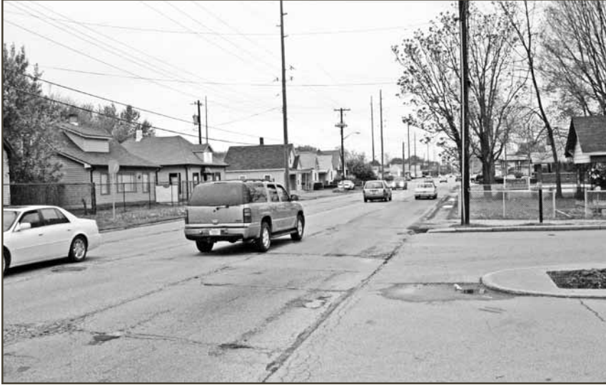
West 30th Street at Alton Avenue
