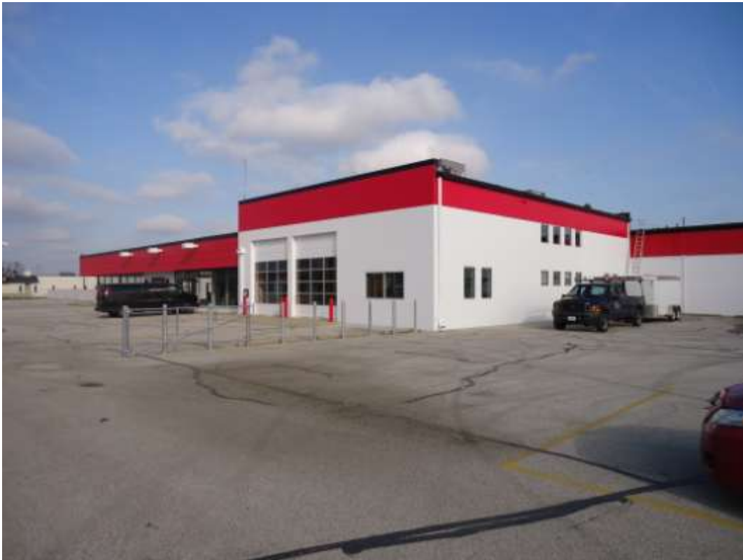
1) Primary structure on site
