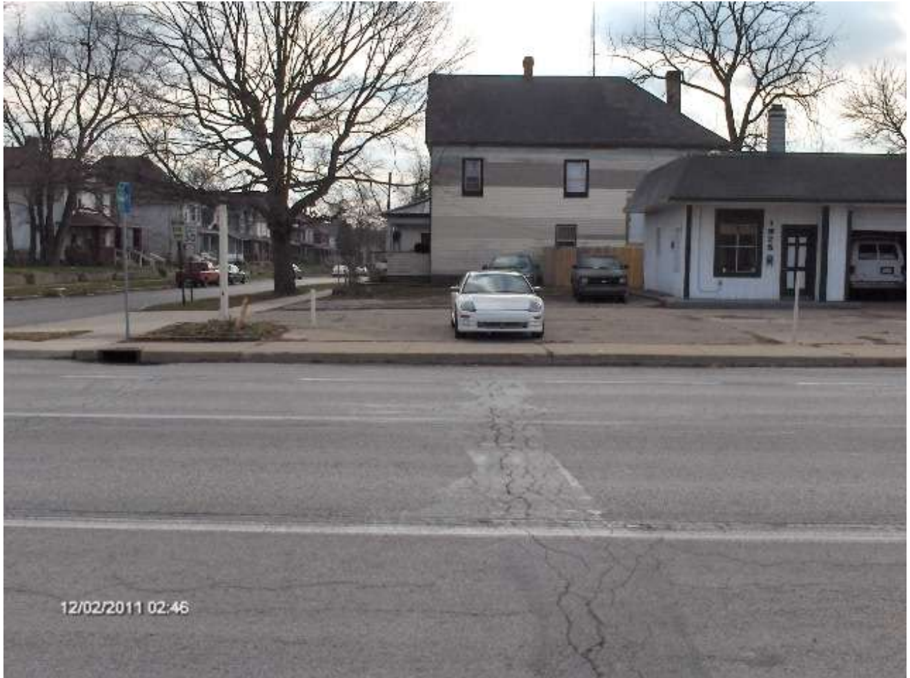
Photograph Four – Proposed eastern curb cut
