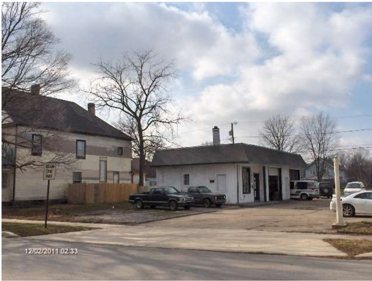
Photograph Two – Randolph Street Curb Cut
